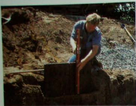
Sidewall supports need to be levelled to a perfect vertical alignment.
