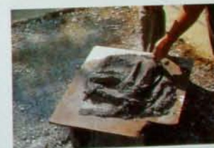
Mortar is kept nearby.
