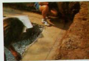
The concrete footing is marked to guide in block placement.
