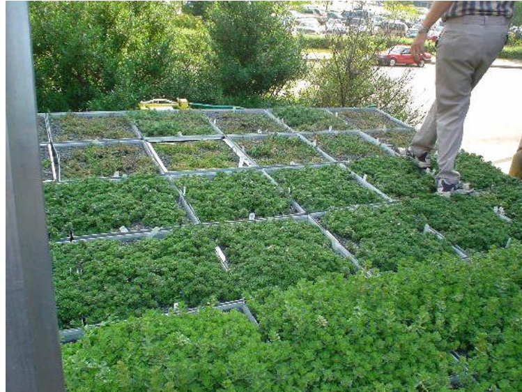
Figure 3.2 Photograph showing Green Roof Block System (Adapted from St. Louis Metalworks Company)
