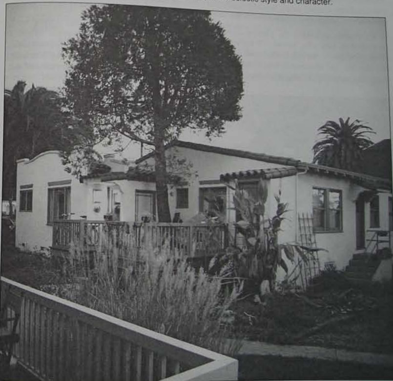
Photo 8.5: A pre-existing building refurbished as a duplex of eclectic style and character.
