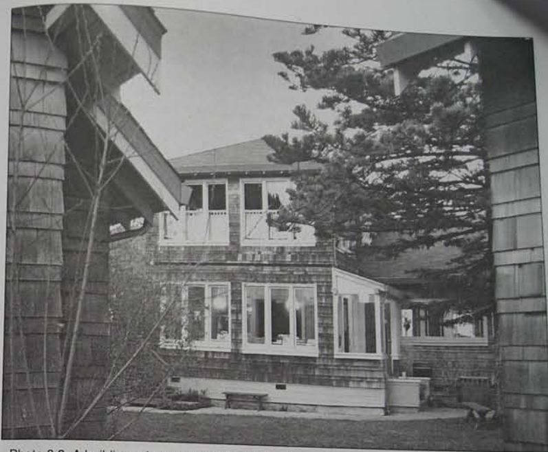
Photo 8.3: A building refurbished as the common house (downstairs) and an apartment (upstairs).
