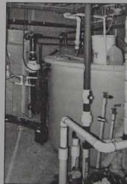
Photo 2.5: Grey water system. Photo 2.6: Recycled window.
