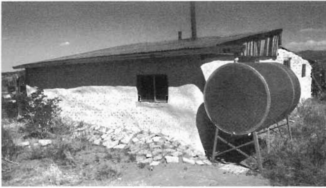
Fig. 3.38. The Howells' home and 500-gallon (1,895-l) galvanized steel cistern
