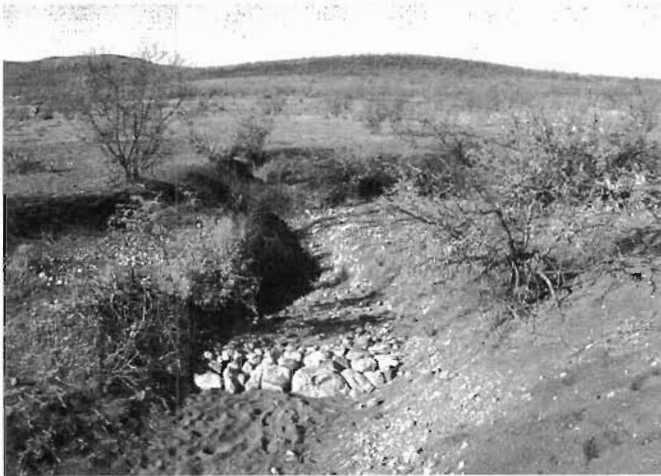
Fig. 3.25A. One-rock check dam, Red Windmill Draw, Malpai Ranch, near Douglas, Arizona. One-rock dams are just one rock high and placed in three to five parallel rows packed tightly together across the drainage. There is no apron. Reproduced with permission from An Introduction to Erosion Control by Bill Zeedyk and Jan-Willem Jansens. Photo credit: Van Clothier of Stream Dynamics. For color photo see inside front cover.
