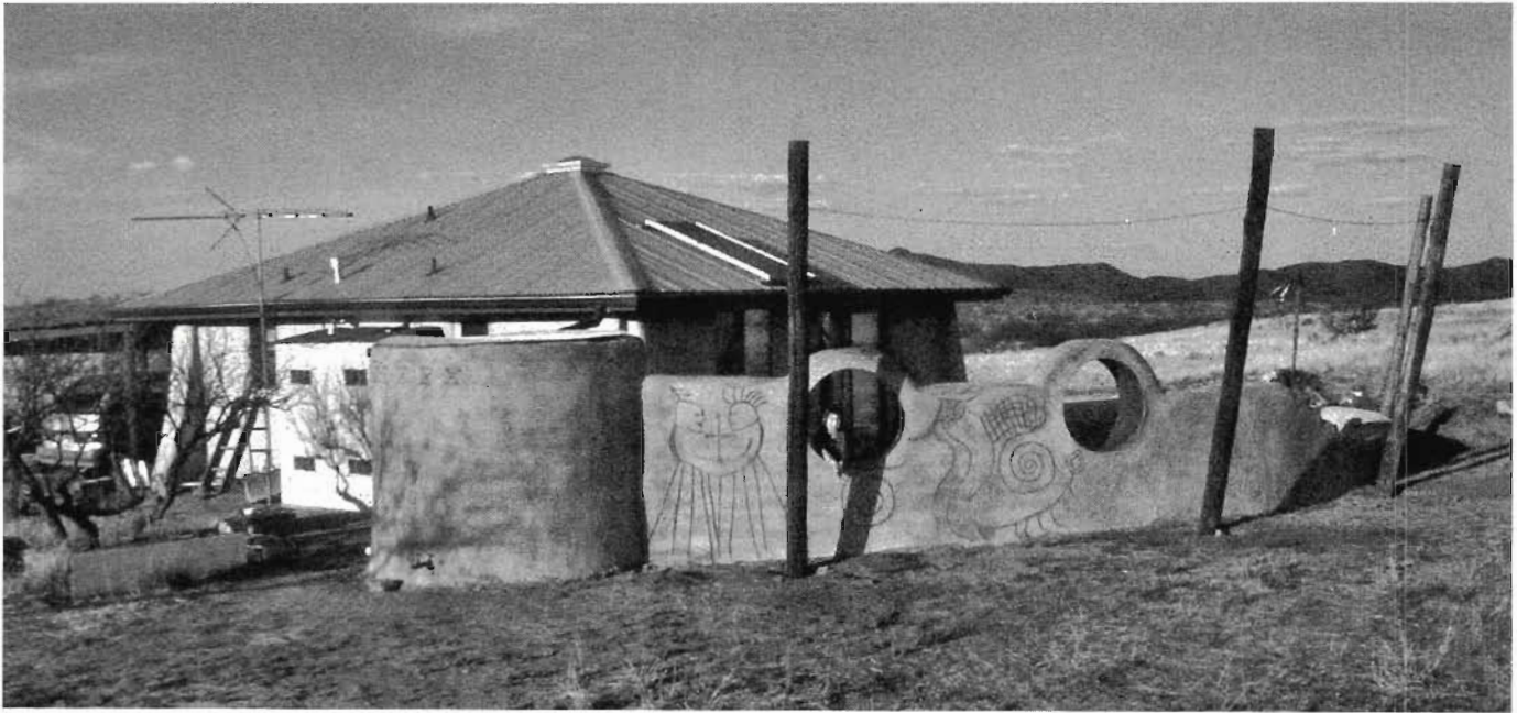
Fig. 4.13. The prevailing wind's view of Allegra Ahlquist's cistern and wall, creating a protective sun trap and windbreak for her courtyard. Solar panels on roof faces south.
