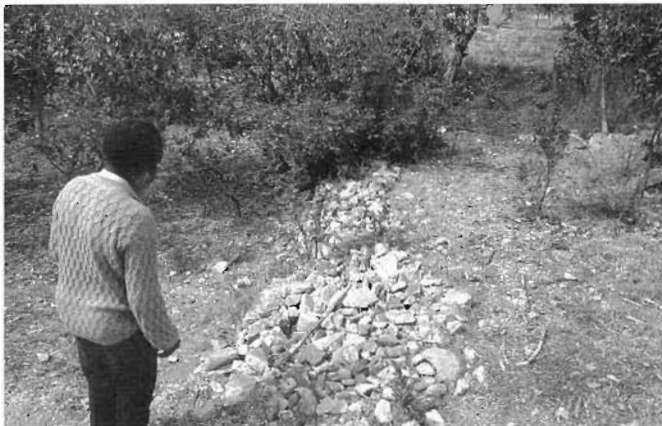
Fig. 1.5. A loose-rock check dam that has healed a once-erosive gully
