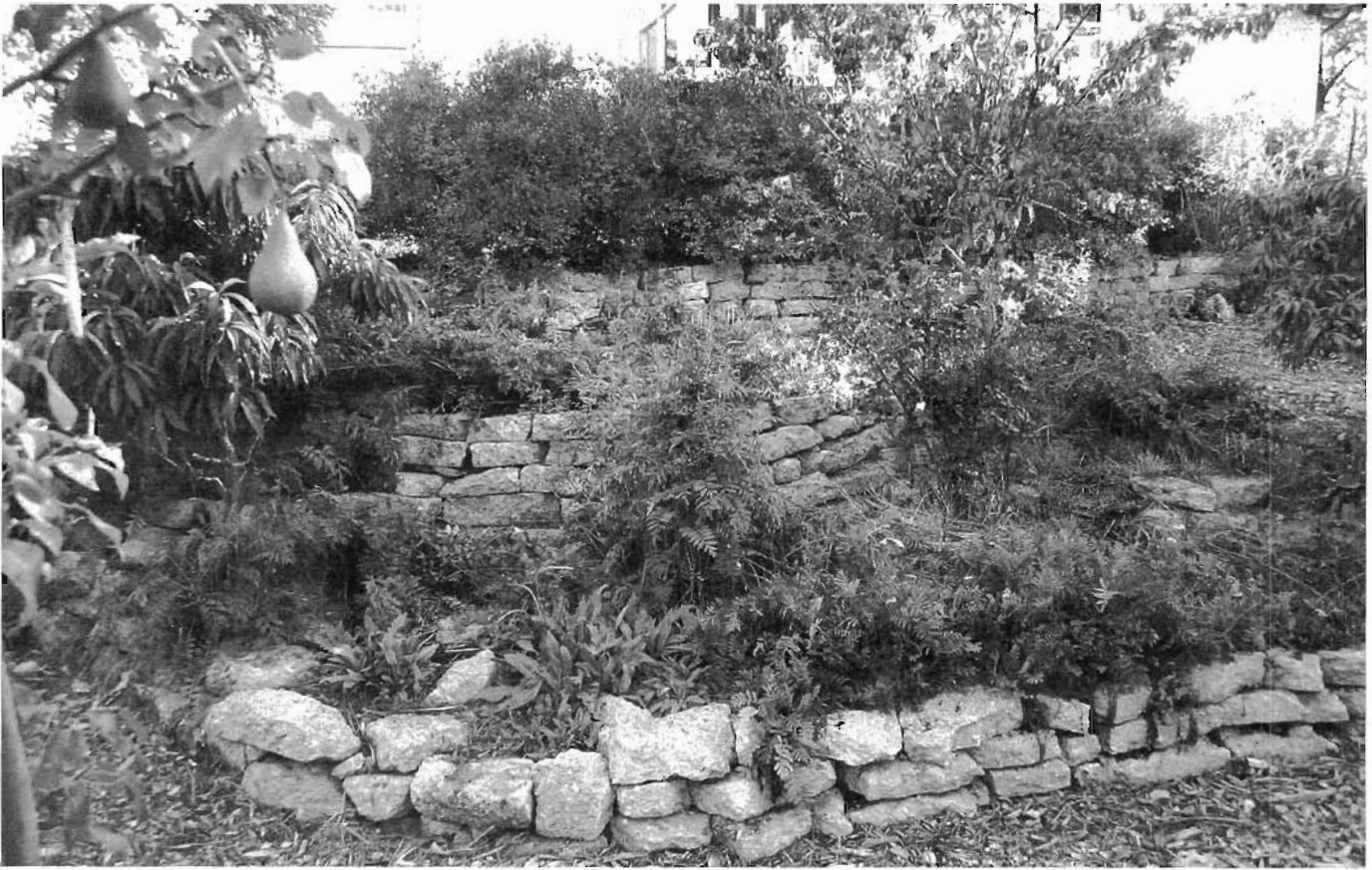
Fig. 3.5. Terraces stabilized with salvaged concrete retaining walls in the sloped backyard at the Zemach residence, Los Alamos, New Mexico. For color photo see inside back cover.
