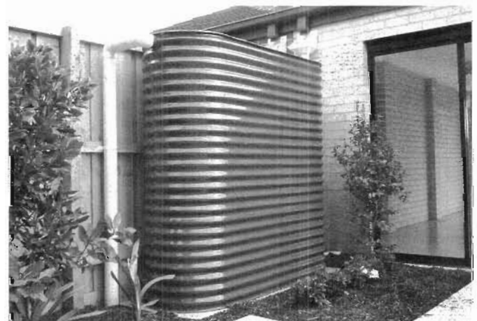
Fig. 3.33. A 300-gallon (1,136-liter) corrugated steel WATERHARVEST SLIMLINE® tank. Reproduced by permission of BlueScope Water. Slim tanks work great for small spaces and narrow yards, and are available up to a 1,500-gallon (6,000-liter) capacity in metal, plastic, or fiberglass. They can double as garden walls or privacy screens.
