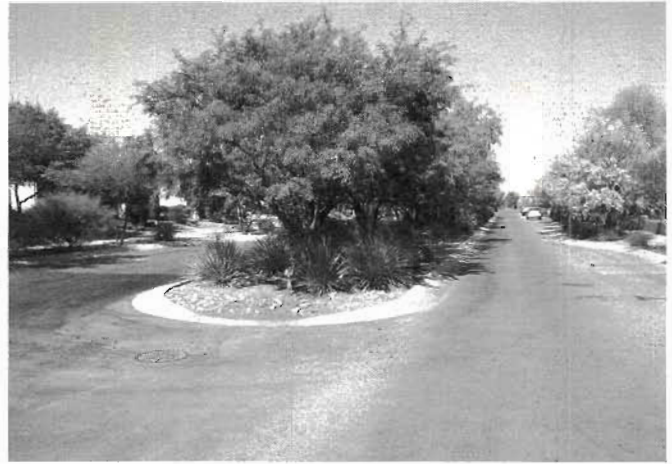
Fig. 3.17. Narrower streets and young native food-producing mesquite trees irrigated by harvested street runoff, Civano, Tucson, Arizona
