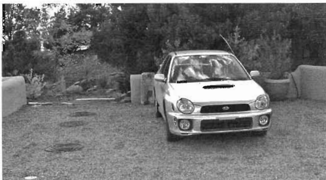
Fig. 3.35. A below-ground 1,200-gallon (4,542-liter) concrete cistern engineered to take weight of vehicles above. Only access lids are visible. Cistern collects roof runoff from home. Santa Fe, New Mexico
