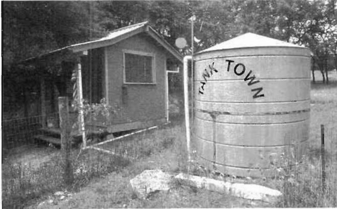
Fig. 3.30. Galvanized tank and wet system downspout, Tank Town, Texas. A wet sysem downspout pipe always has water in it so it cannot be used in cold climates. The horizontal run of pipe is supported by the soil, and then rises up (but not higher than its inflow point at the gutter) to enter a tank or earthwork.
