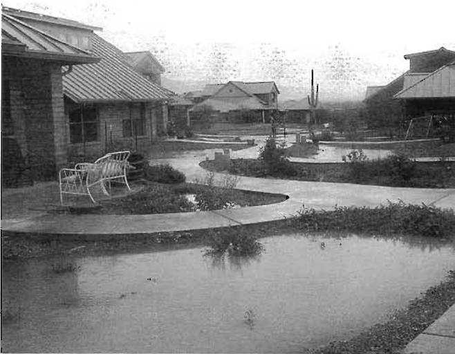
Fig. 3.11A. Rainfall collected in newly constructed infiltration basins minutes after a large summer storm. The basins have not yet been mulched or planted. Milagro Cohousing, Tucson, Arizona Credit: Natalie Hill. For color photo see inside front cover.
