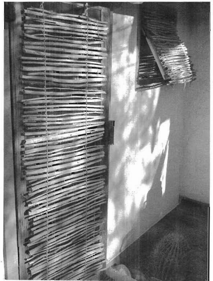
Fig. 4.9. East-facing exterior blinds doubling as pollinator habitat. Beneficial carpenter bees live in the hesperaloe flower stalks of which the blinds are made. Note dappled shade from trees to east provides additional cooling!
