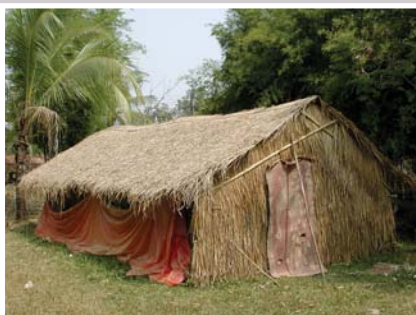
Figure 30. This growing house has its whole sides covered with Imperata grass to prevent flies.
