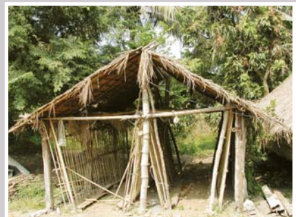
Figure 32. Rack frame structure
