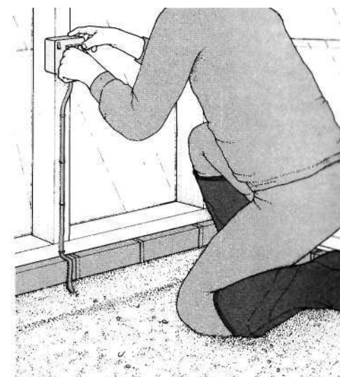
4 Connect the soil heating cable to a thermostat, if one is supplied with the cable kit, or direct to an outlet. Carefully follow the maker's instructions on installation.
