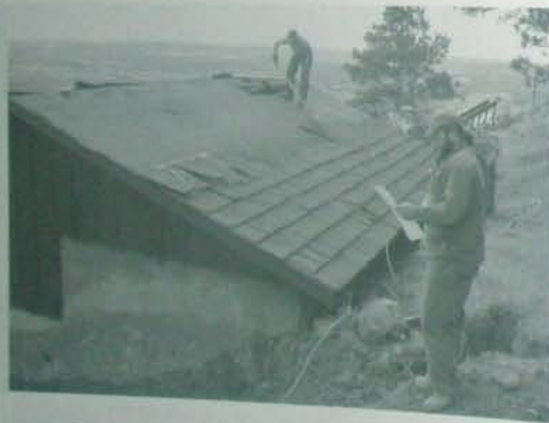
Fig. 1.4: Roof deconstruction. Credit: David Johnston.
