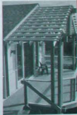
Fig. 1.14: The deck and trellis. Credit: Kim Master.
