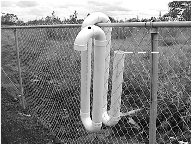
An overflow device that will keep the water level as indicated. The pipes on the near side of the fence hang outside the tank. In this design, a hole must be made on the top of the pipe in the foreground for the system to function properly. If a T joint is used instead of an elbow, the hole is not needed.
