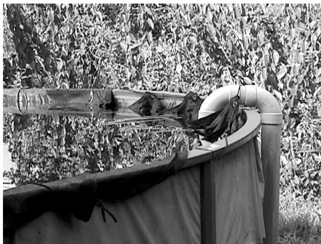
Sagging and broken covers like this one are very common. The storage tank is where water sits the longest, and keeping it covered is important to reducing water contamination.
