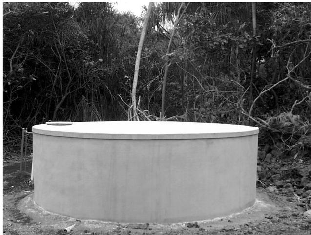
Ferroconcrete tanks, also known as ferrocement tanks, are new to the local market and growing in popularity. Like solid concrete tanks, they can be designed into a home's structure.
