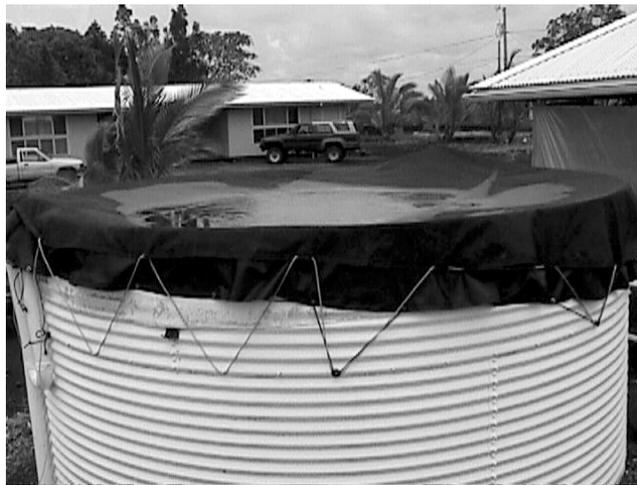
Mesh covers often sag into the water when the tank is full or the mesh stretches in the sun. The resulting puddle attracts birds, insects, and debris, which contaminate the water.
