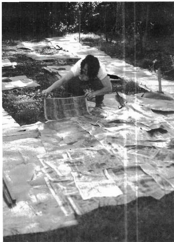
FIGURE 6.19. In this sheet-mulch project we were short on mulch materials, so we put no mulch under the weed barrier. We used newspaper under the growing beds because the existing weeds were few and easily smothered. Wetting the newspaper before laying it prevents wind-lift. Lay the sheets like shingles from one side of the space to another, always leaving the same edge free each time you lay a piece. This allows you to throw on the next mulch layer like rain, so the mulch presses the seams closed to seal out weeds. Use at least six sheets of thickness, and at least 4 inches (10 cm) of overlap at the seams, more if possible. Photo by Dave Jacke.
