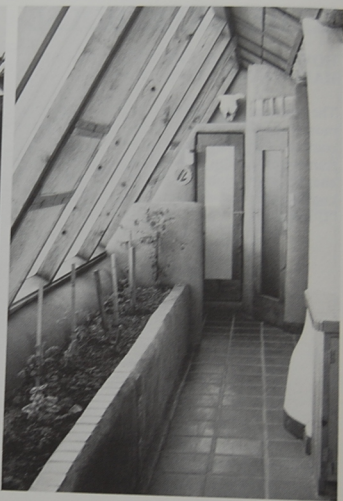
Finished Greenhouse - interior.
