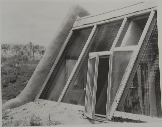
Finished Greenhouse - exterior.
