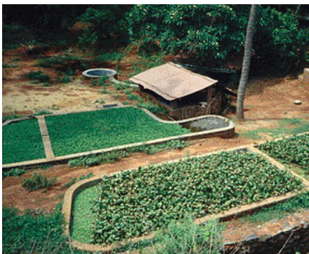
Figure 4: Sewage system using water hyacinth ©Paul Calvert/Practical Action
