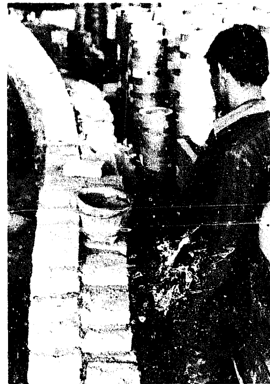
Fig. 2-86: Stretcher courses in a Chinese-type tube kiln
