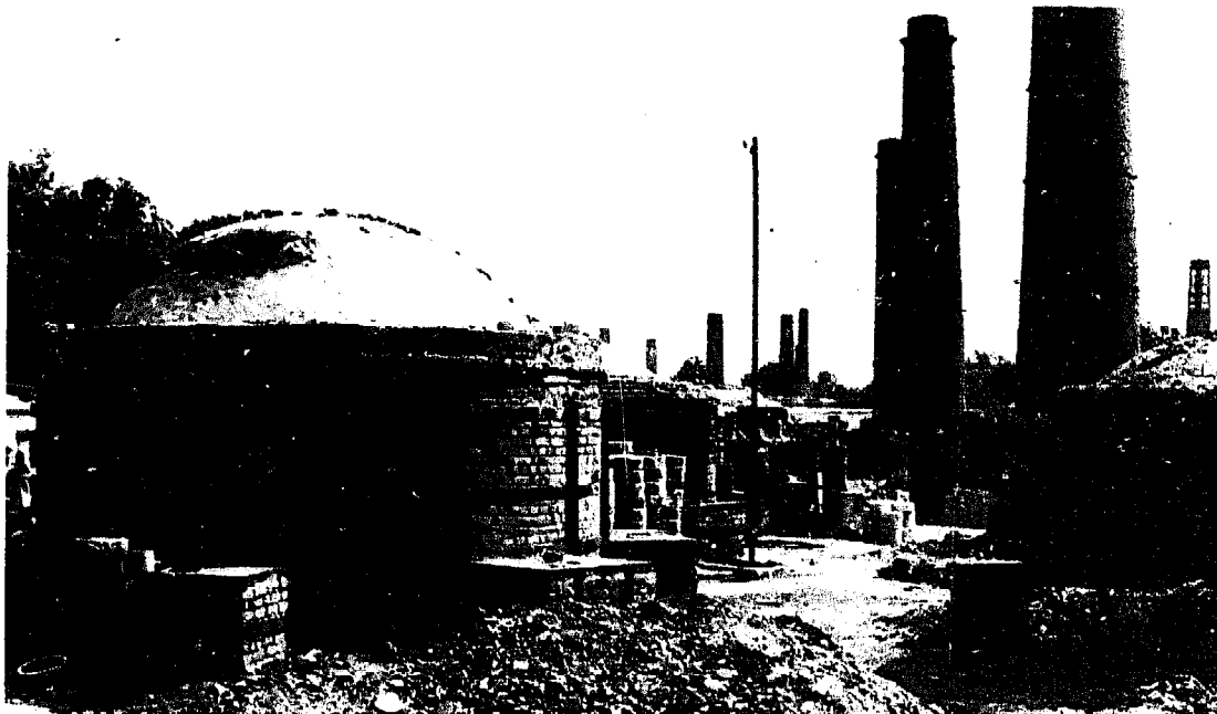
Fig. 2-18: Circular coal-fired down-draught kiln. Khurja, India.
