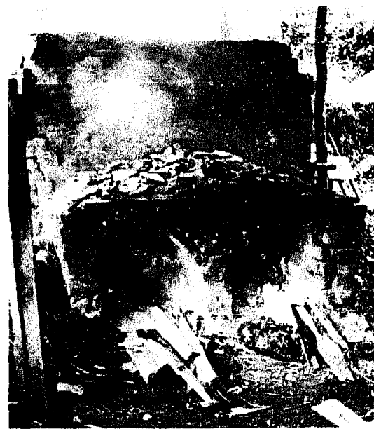
Fig. 2-132: The fire is in this case kept outside the firebox until the water smoking period is over.
