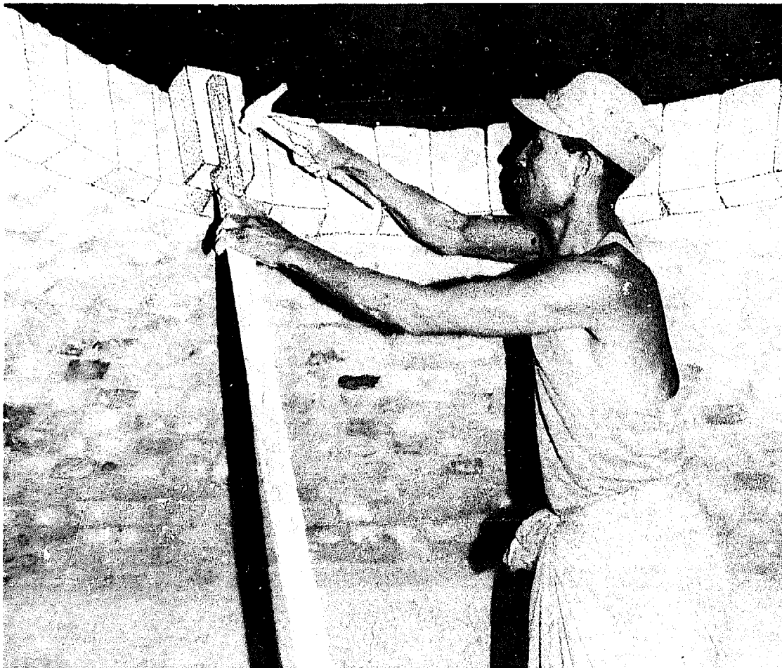
Fig. 2-98: Construction of a dome
