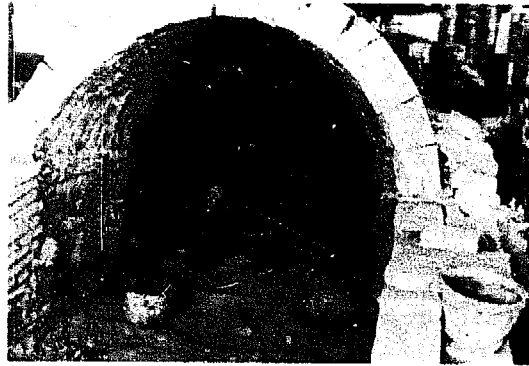
Fig. 2-28: Saggars set in a tube kiln under repair
