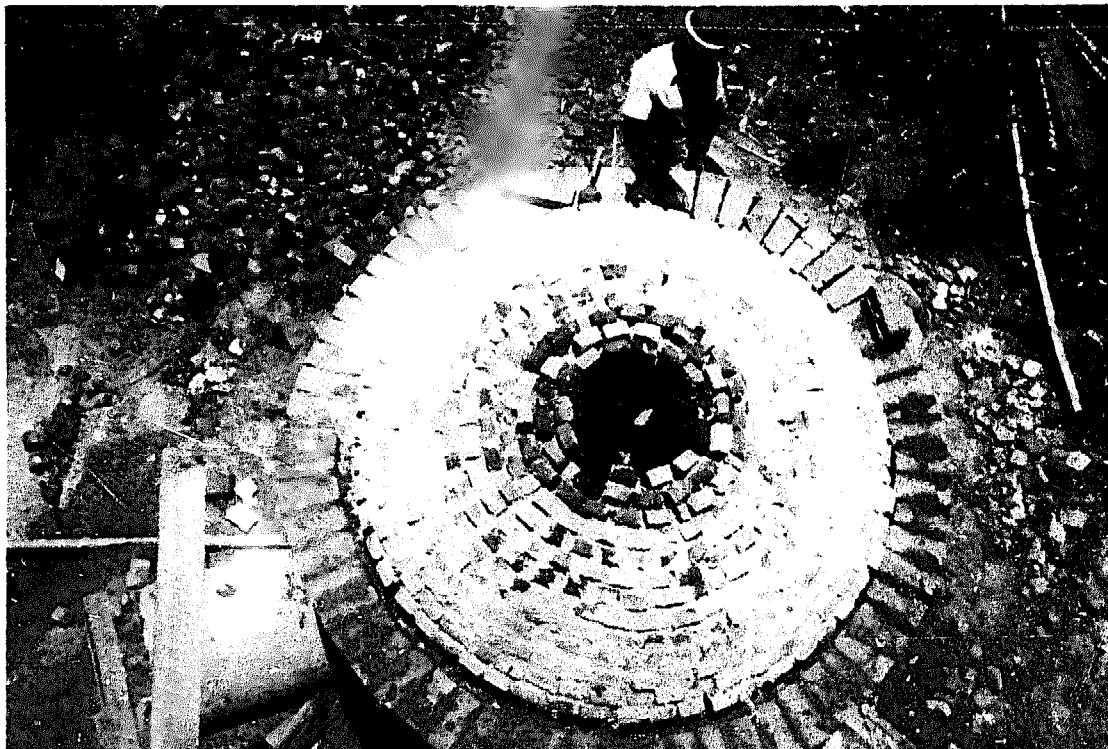
Fig. 2-102: Only a few courses are still to be laid and each brick has to be cut to size.
