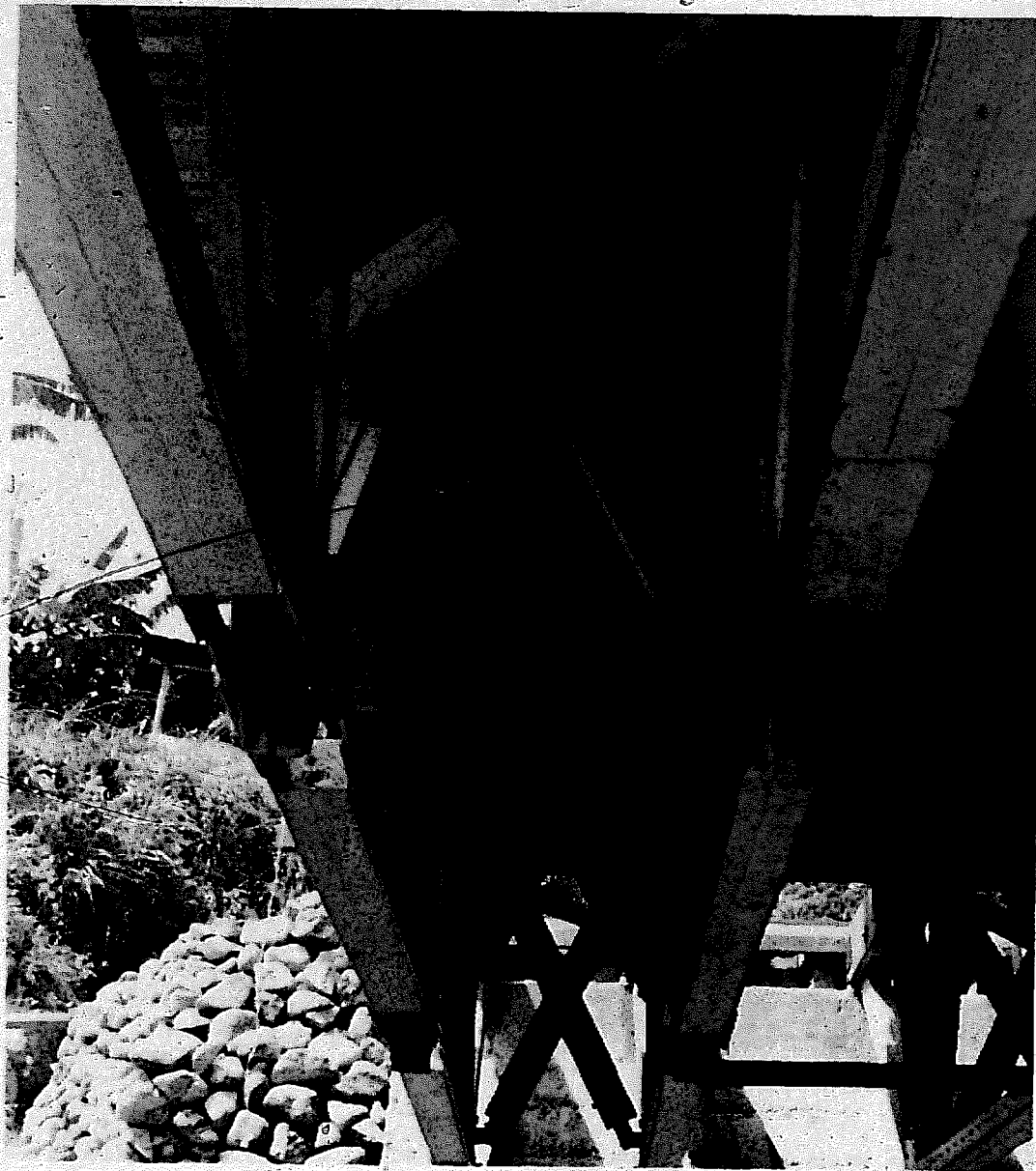
Cross and diagonal bracing on underside of bridge, Honduras
