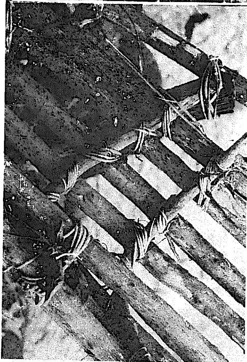
Fig. 79 Lashing using stripped cane, Sau River Bridge.
