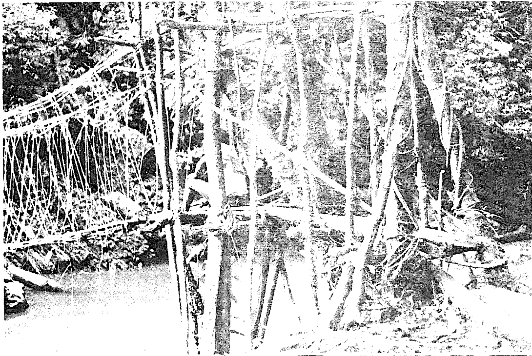
Fig. 123 Anchorage and approach, Iamdelmin Bridge.
