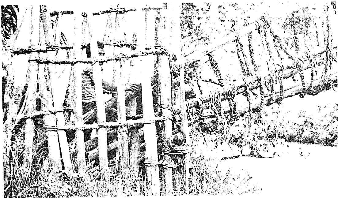
Fig. 74 The south abutment, looking west, Kopeme Bridge.
