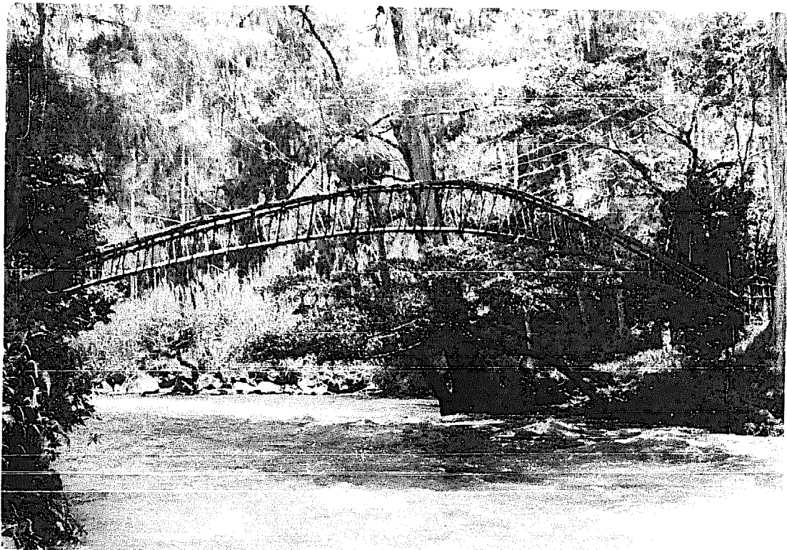
Fig. 59 Kubib Bridge over Mendi River, seen from the east bank looking south.
