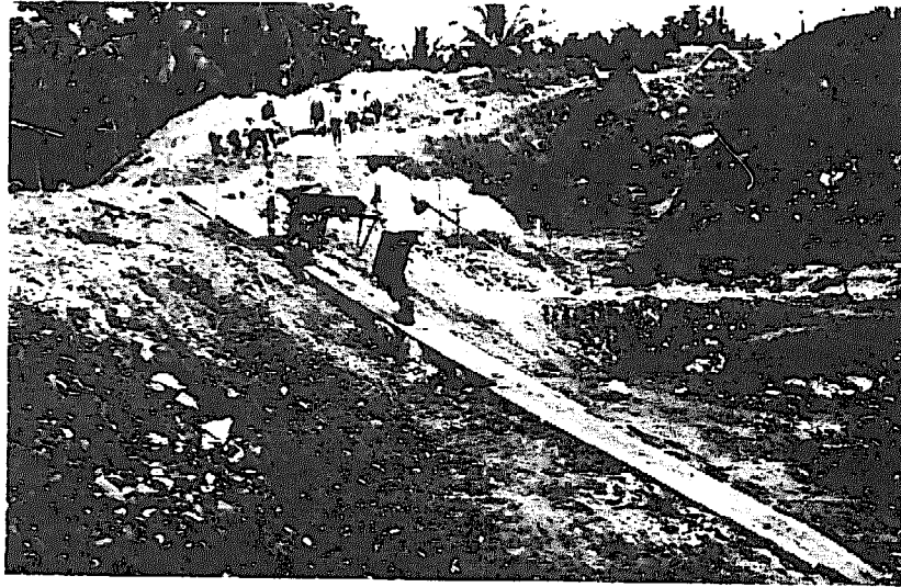
Figure 3. HAULAGE ON UP-GRADE USING WESTERN-STYLE WHEELBARROW AND TIMBER BARROW RUN (Weight 16kg Payload 75kg)
