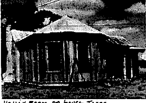
1/2 Hex Room on house, Texas
