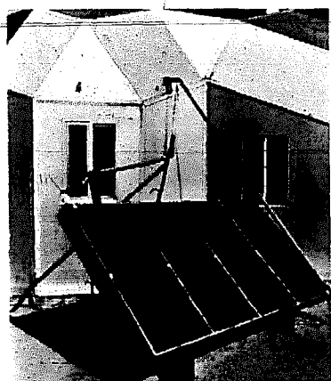
SOLAR WATER HEATER
