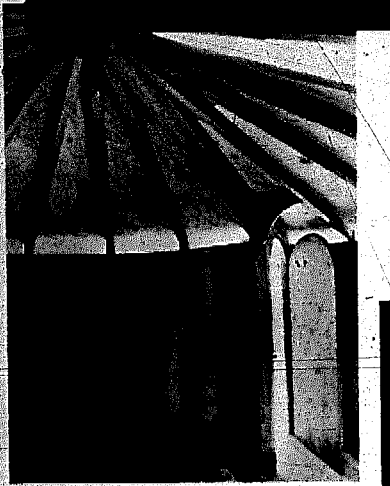
This spiral building evolved its shape as it was being built. Starting with the floor of a water tower, the builders decided to extend it to an oval, then egg shape. When they thought about fitting in a door, the nautilus shell spiral came about. It was built as a zendo, by Bob Anderson. Hyperbolic paraboloid shelter with eucalyptus poles and plywood. There are no walls. By Barry Smith.
