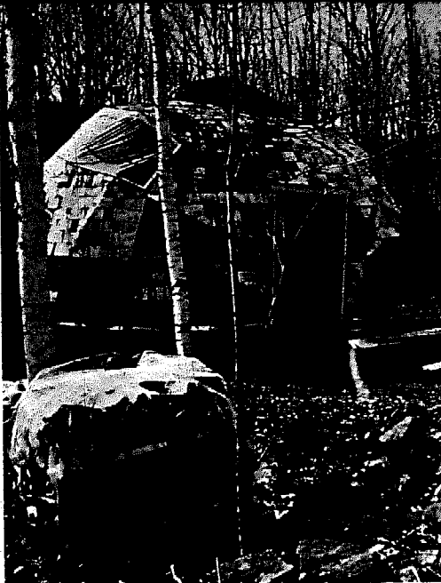
DOME SHINGLED WITH ALUMINUM PHOTO OFFSET PLATES
