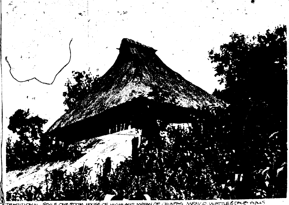
TRADITIONAL STYLE ONE-ROOM HOUSE OF HIGHLAND MAYAN OF CHIAPAS, MEXICO. WATTLE & DAUB WALLS
