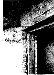
FRAME ON ADOBE WALL
