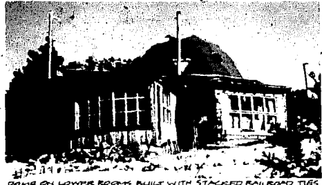
DOMES ON LOWER FLOORS BUILT WITH STACKED RAILROAD TIES.
