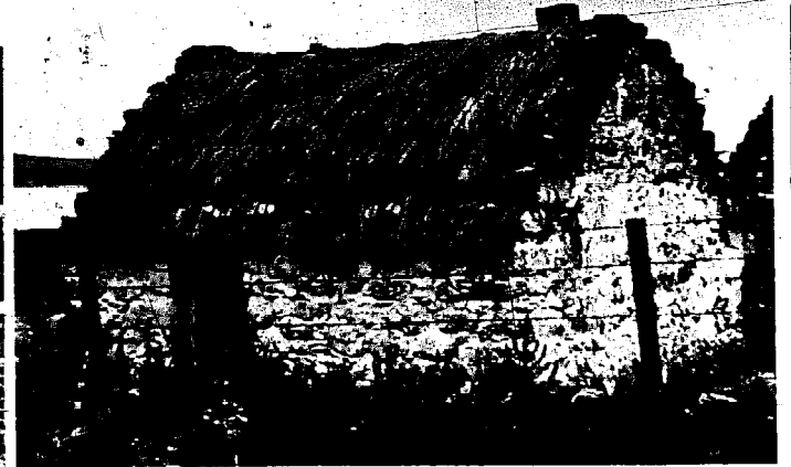
SIMPLE IRISH THATCHING METHOD. ROPES HOLD STRAW DOWN. HORIZONTAL ROPES WEIGHTED BY ROCKS ON EITHER SIDE.
