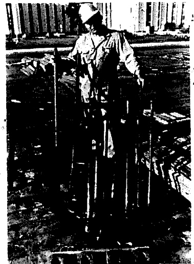
GEORGE'S TOOLS FOR THE PRO, STEEL SAWHORSES THAT CAN HOLD 2000 BOARD FEET OF LUMBER, AND SPECIAL TOOLS TO STRIP 1x6, 1x8, 1x10'S WITHOUT BENDING OVER. TWO BIG BARS OF CHROME MICAL STEEL THAT CAN BUST CONCRETE.
