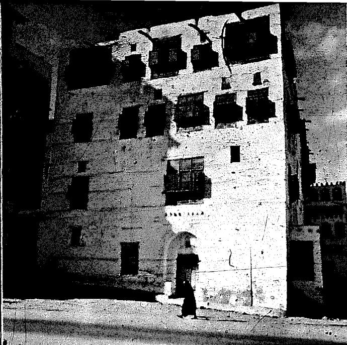
ADOBÉ BRICK AND PLASTERED APARTMENT BUILDINGS JEDDAH, SAUDI ARABIA
