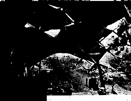
This spiral building evolved its shape as it was being built. Starting with the floor of a water tower, the builders decided to extend it to an oval, then egg shape. When they thought about fitting in a door, the nautilus shell spiral came about. It was built as a zendo, by Bob Anderson. Hyperbolic paraboloid shelter with eucalyptus poles and plywood. There are no walls. By Barry Smith.
