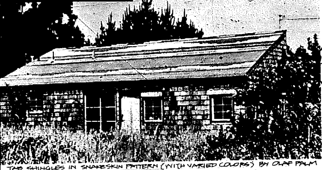
TAB SHINGLES IN SANDSKIN PATTERN (WITH VARIED COLORS) BY CLAF PALM
