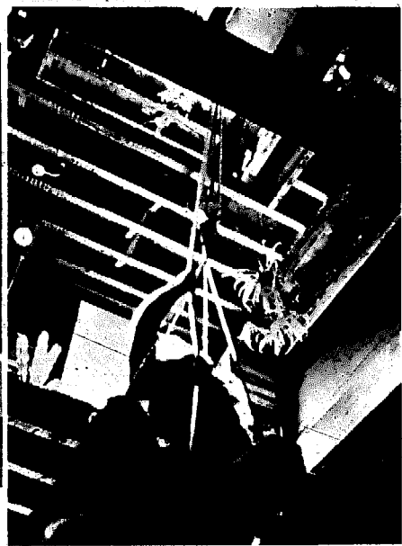
CENTRAL SHAFT CUT THRU 4 FLOORS AND SKYLIGHT INSTALLED IN ROOF. HAND POWERED OAK CHAIR ELEVATOR.
