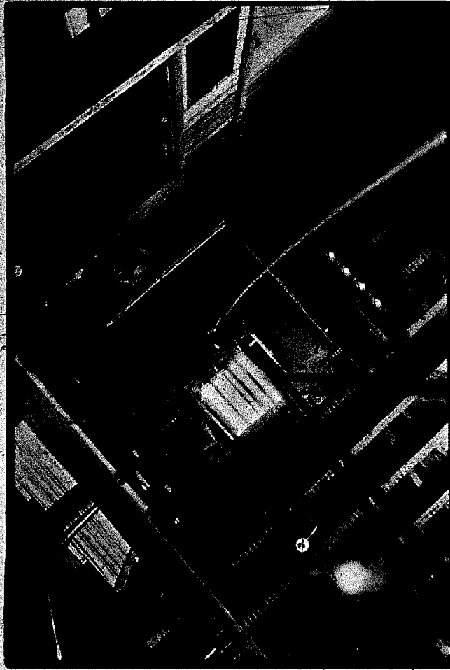
CENTRAL SHAFT CUT THRU 4 FLOORS AND SKYLIGHT INSTALLED IN ROOF. HAND POWERED OAK CHAIR ELEVATOR.
