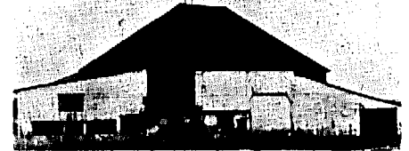
Polygonal barn in Quebec, an extended octagon with lean to's added on
