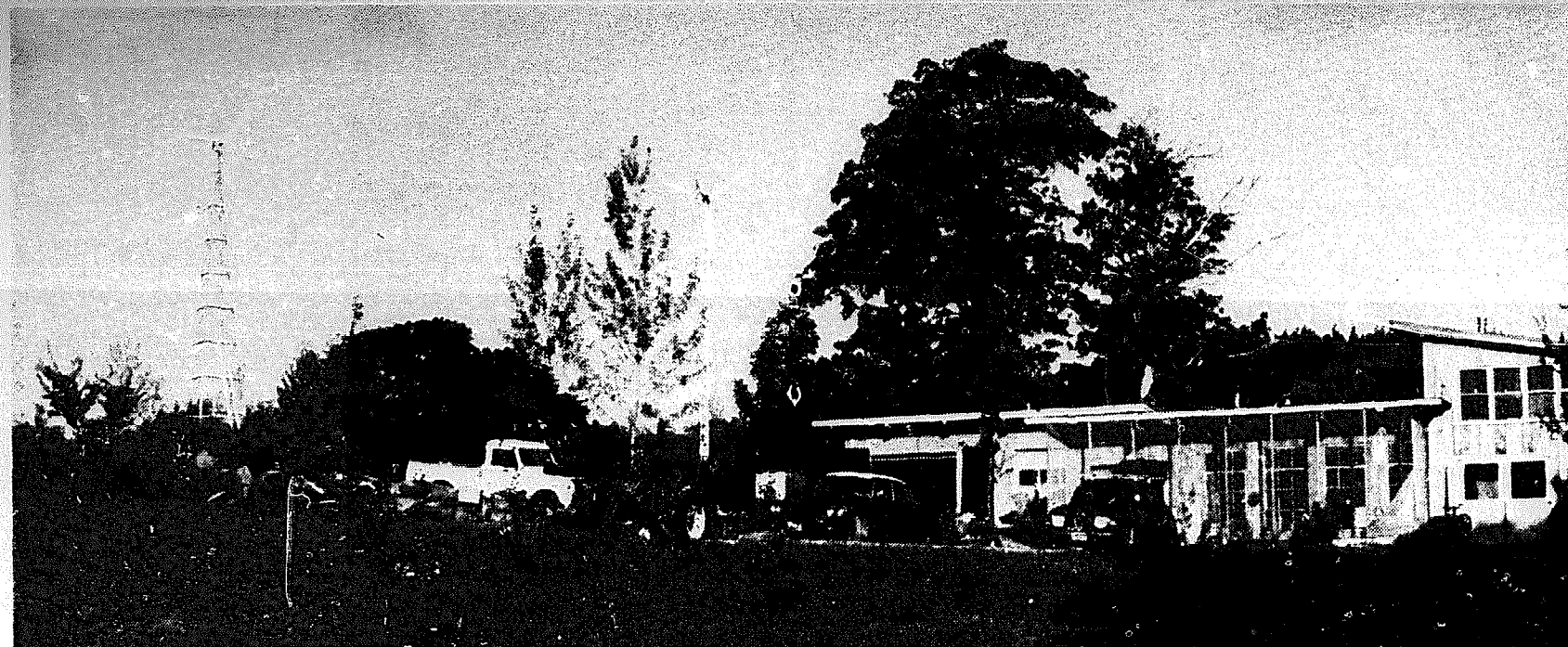
Our wind-powered homestead, summer 1974. Dunlite 2000-watt left, Elektro 6000-watt center.
