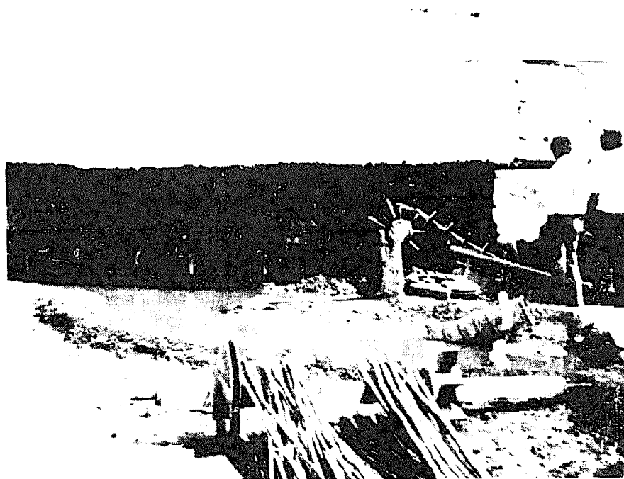
FIG. 1. A Six-Sail Thailand Windmill as Used in the Salt Works (Bare Poles Condition)
