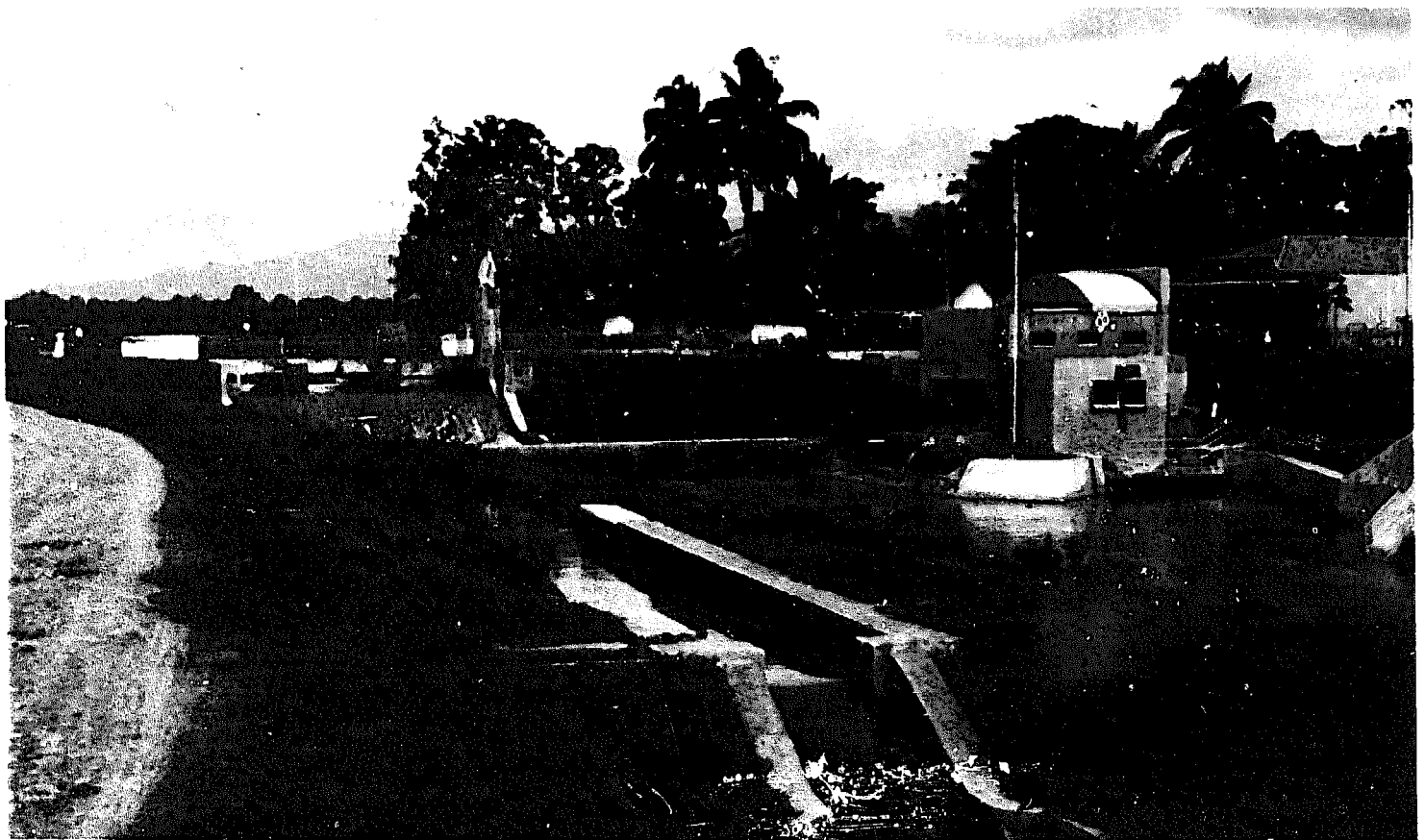
WONODADI, INDONESIA Low-head, 210 kW installation at a drop on an irrigation canal.
