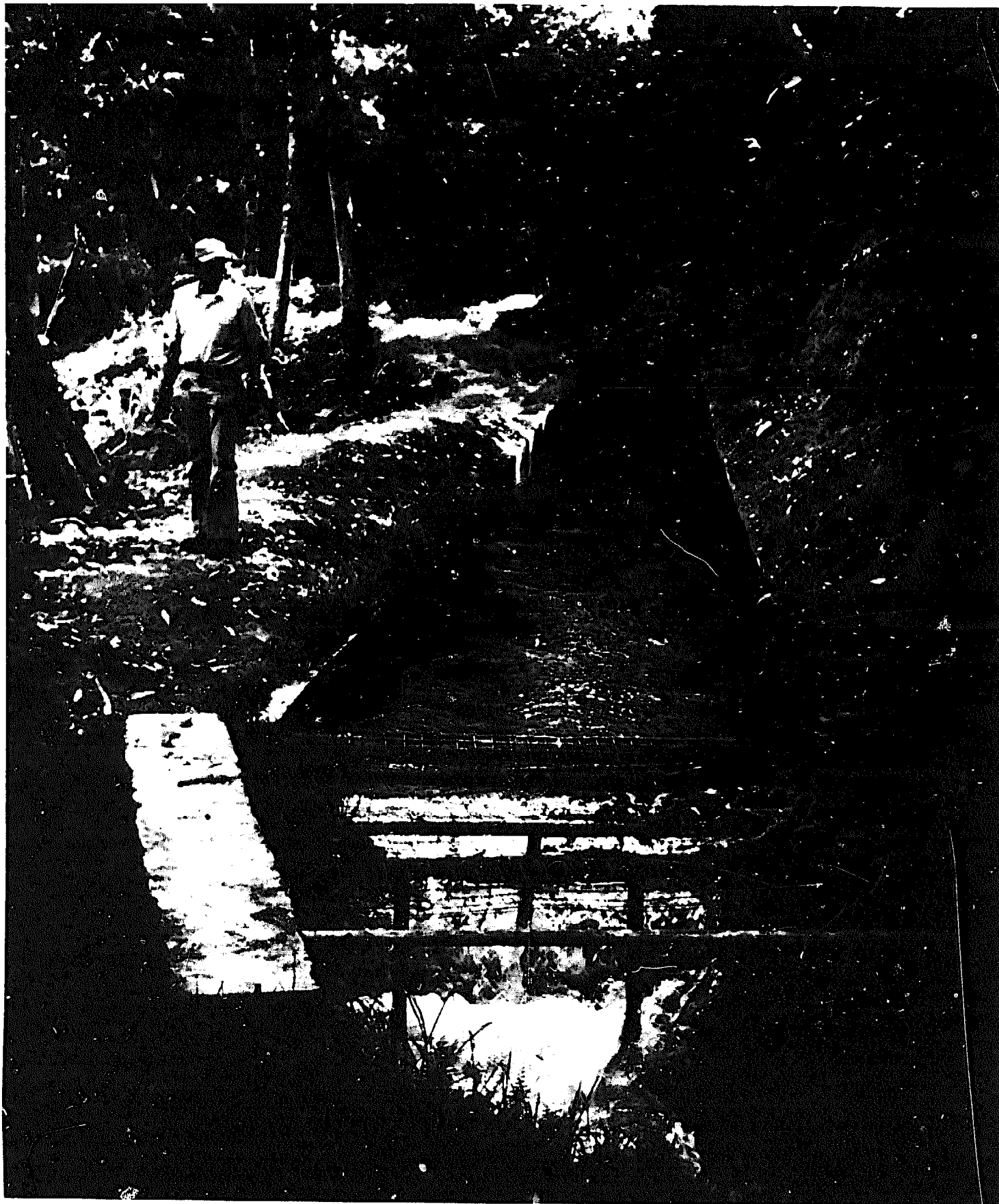
KUDJIP, PAPUA NEW GUINEA (90 kW) Intake to the penstock seen at lower left. With no provision made for a forebay for settling, landslides from the slope at the right resulted in excessive wear of the turbine.
