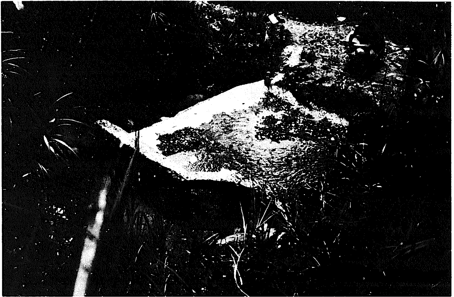
SOPAS, PAPUA NEW GUINEA Intake trashrack facing slightly downstream toward the crest of the weir in order to avoid rainy season floods.
