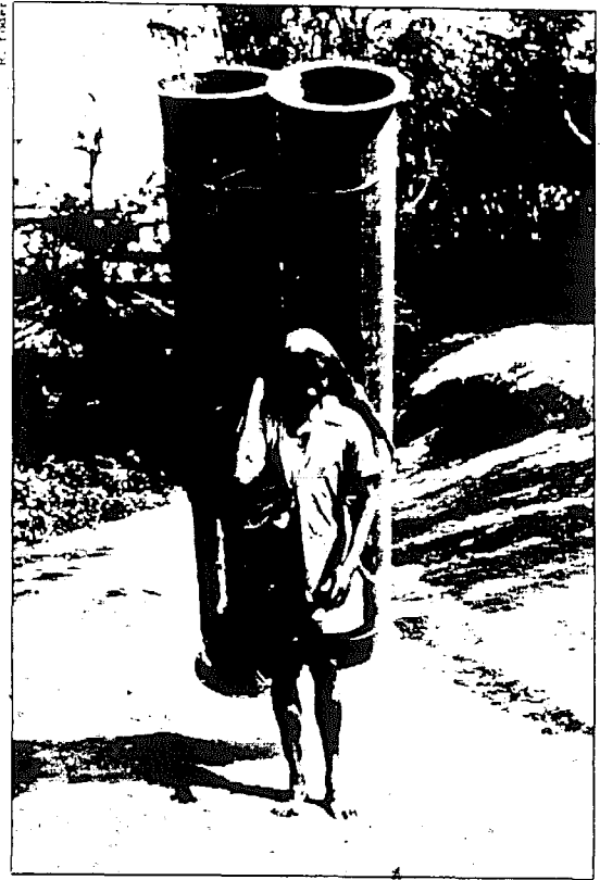
Fig. 27. After the site excavation has been completed and the equipment fabricated at Butwal, porters carry the necessary materials to the site. The two sections of penstock shown weigh about 100 kilograms.
