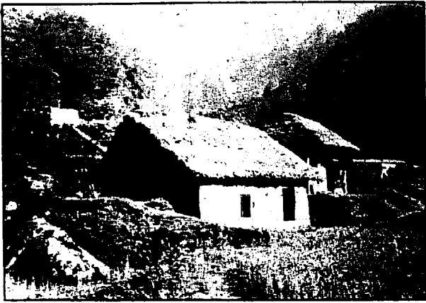
Fig. 21. A mill house with the owner's house in the background. The forebay and penstock can be seen at the left.
