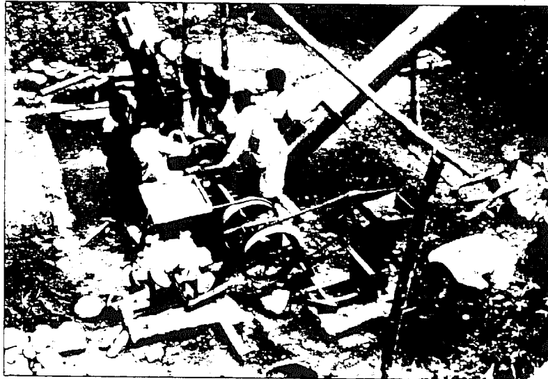
Fig. 31. All the equipment has been aligned and set in concrete.
