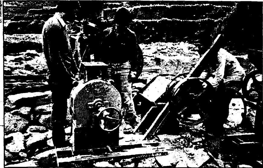
Fig. 17. The new turbines are mounted above the mill floor on a common mounting-frame which is eventually set in concrete. Here the installation team is shown using a string to align the pulleys.
