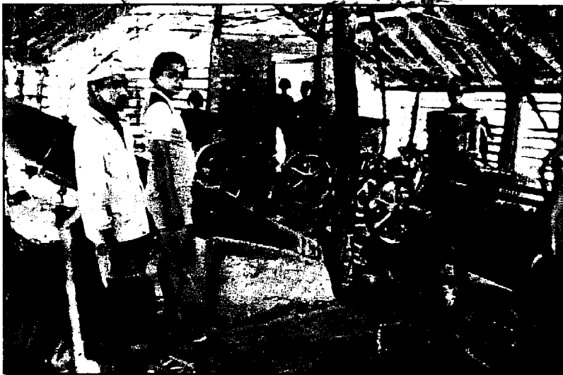
Fig. 15. At Ampchaur, the turbine is placed below floor level.
