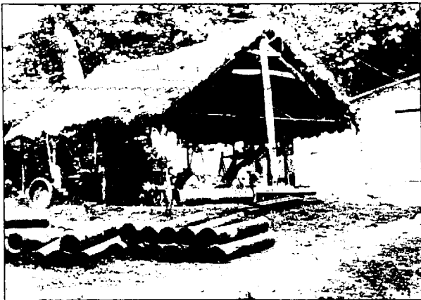
Fig. 11. The test site located at the workshop of BEW. Sections of penstock pipe in the foreground are ready for pressure testing.
