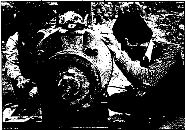
Fig. 40. An installation team securing the flour mill to its base.
