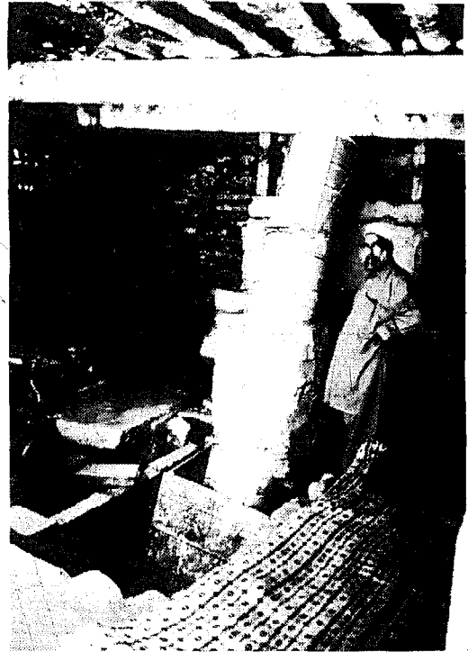
Fig. 17. Oil drum penstock at the Alpuri powerhouse. Operator's bed is in foreground.
