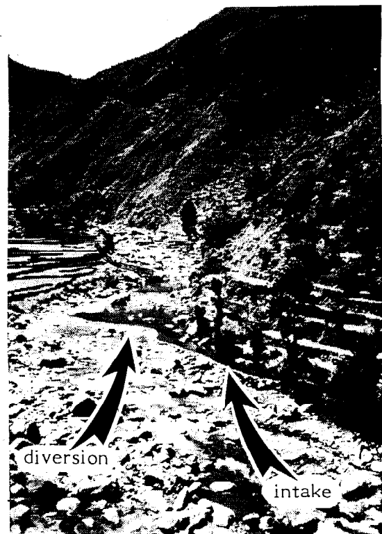
Fig. 4. A temporary structure across the river diverts a portion of the water into an irrigation canal at the right. Similar structures are used with hydropower schemes.
