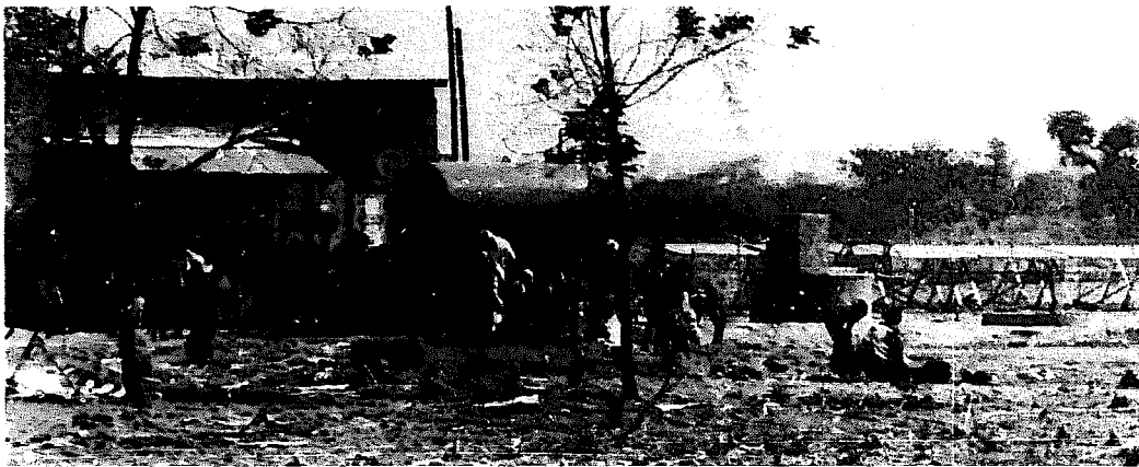
FIGURE 6 A view of the 1.8-kWp solar cell arrays (right center) in the village of Tangaye, Upper Volta, that power a water pump and grain mill. The pump supplies the water-dispensing tank (center). The grain mill, operated as a cooperative by the village, is located in the building behind the tank. This installation, funded by AID and the Government of Upper Volta and under the technical management of the NASA-Lewis Research Center, is intended to explore potential new energy. (Photograph courtesy of NASA-Lewis Research Center, Cleveland, Ohio)
