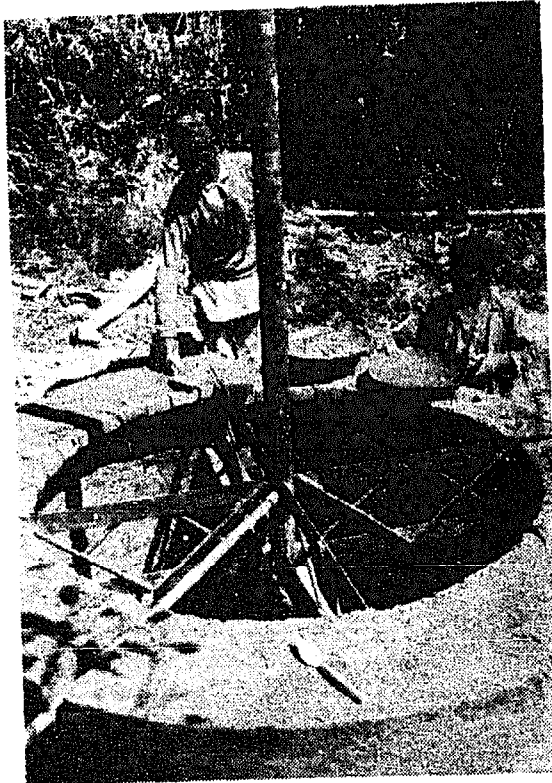
This picture shows the dividing wall in the pit, the fixture of the vertical guide pipe, and the gas outlet.
