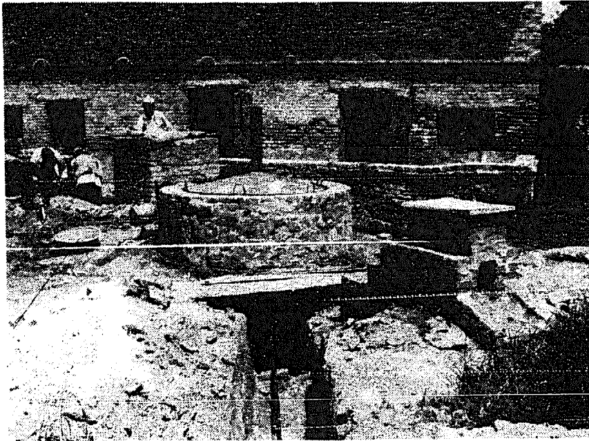
One of the first private gas plants in Kathmandu nearing completion. It is five metres deep and 180 cm in diameter. Notice the mixing trough behind pit, outlet (right foreground) and gas pipe to kitchen.
