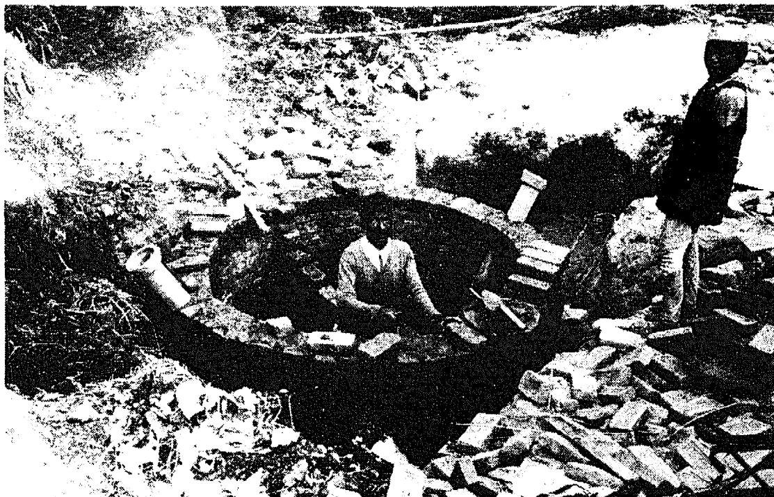
Indian pit design, two chamber construction
