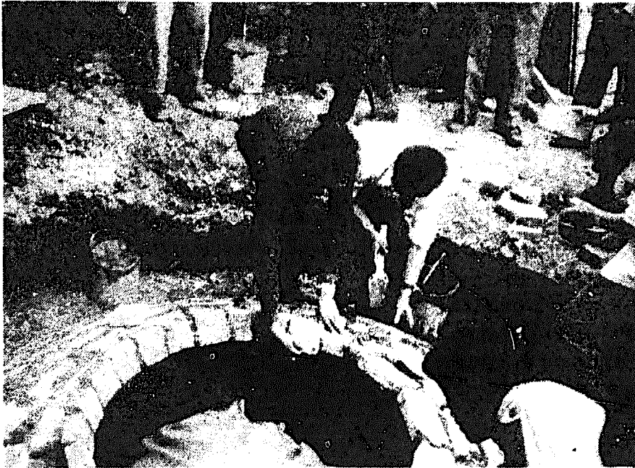
Approaching the manhole. Bricks again vertical, first row half-bricks.
