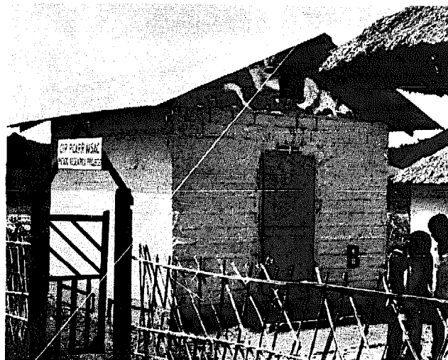
Figure 23. Simple naturally-ventilated stores. A -- Timber, 20 TM capacity (CIP, Huancayo, Peru). B -- Mud-brick or concrete block, 15 TM capacity (CIP-PCARR-MSAC, Baguio, Philippines).
