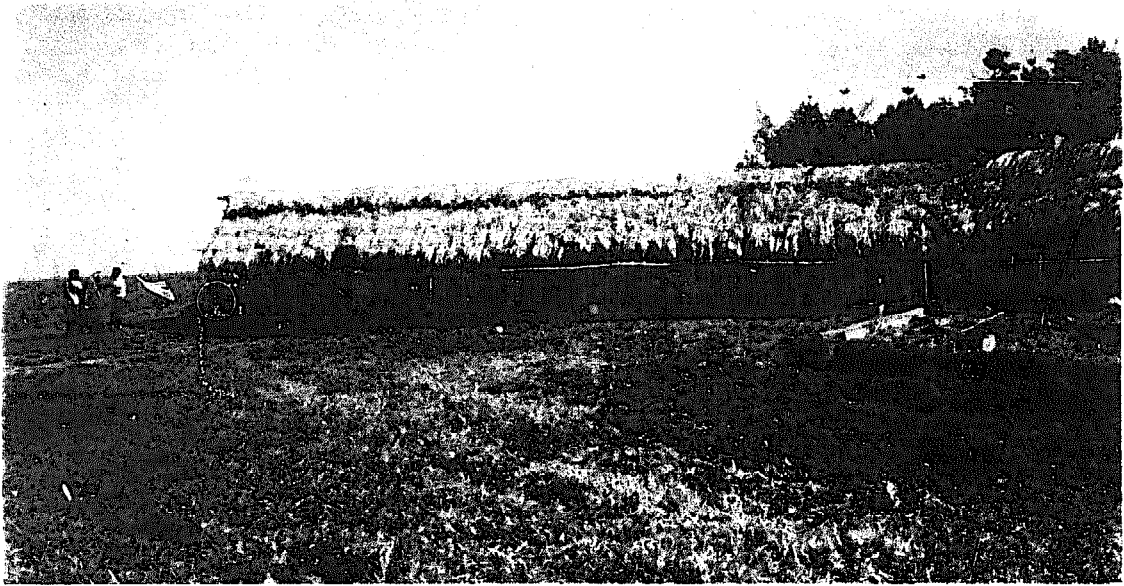
Plate 6. A bush materials piggery in Papua New Guinea. This house has been built on the side of a hill so drainage is not a problem. The hole in the ground in front of the house is to collect the manure and water from the pens and to store it for future use in vegetable gardens.
