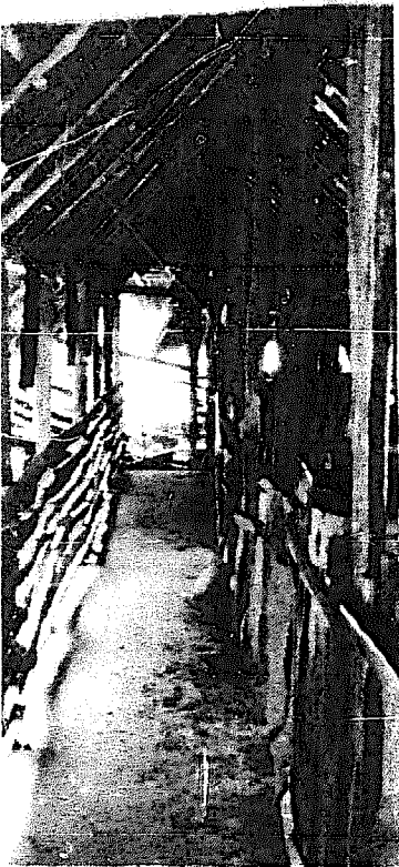
Plate 7. An inside view of a bush materials house. The passage makes the movement of pigs from pen to pen much easier and because it is covered it is a comfortable place for the farmer to work in.
