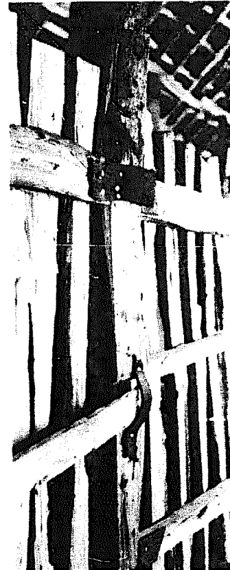
Plate 7. An inside view of a bush materials house. The passage makes the movement of pigs from pen to pen much easier and because it is covered it is a comfortable place for the farmer to work in.
