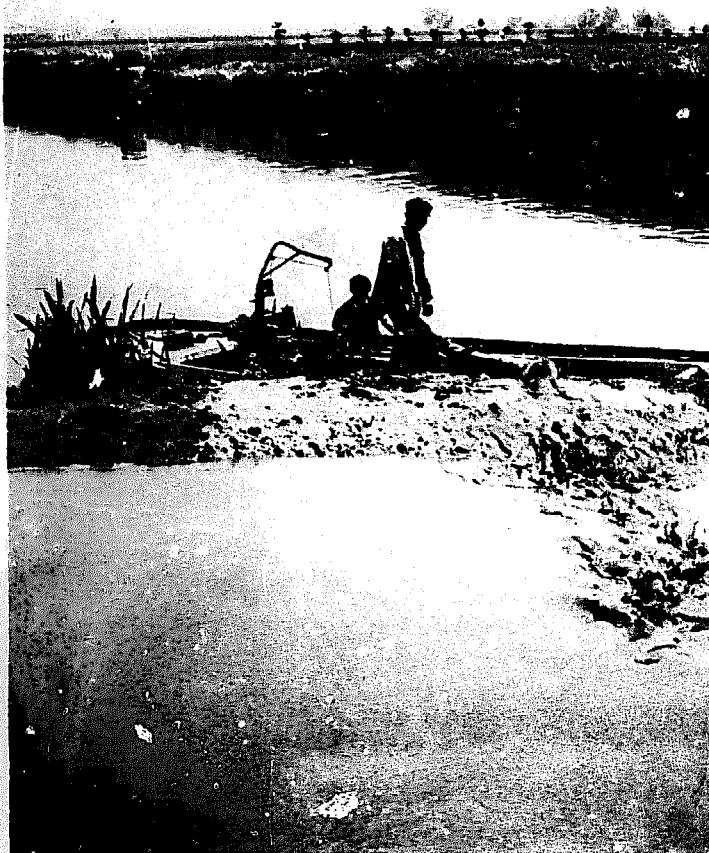
Fig. 6 Boat for sucking silt from the bottom of the canal. Foreground: Silt tank. Malu People's Commune, Shanghai
