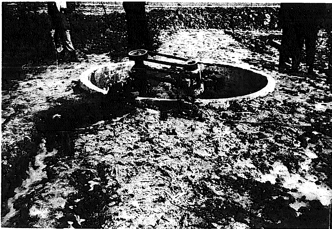
Fig. 46 Outlet of large size bio-gas plant. Effluent pumped into irrigation drain. Cheng Hsiang Production Brigade, Jiangsu Province.
