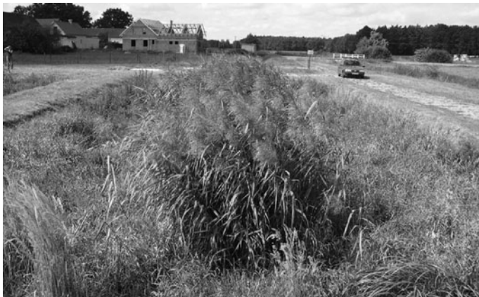
Fig. 11.1 Constructed wetland Břehov. Phragmites band in the middle, in between Phalaris bands. Photo Jan Vymazal
