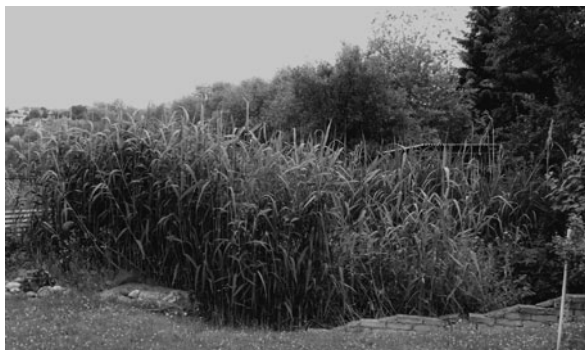
Fig. 13.2 Example of on-site constructed wetland for 4 PE. Kostelec nad Černými lesy, Czech Republic. Photo author
