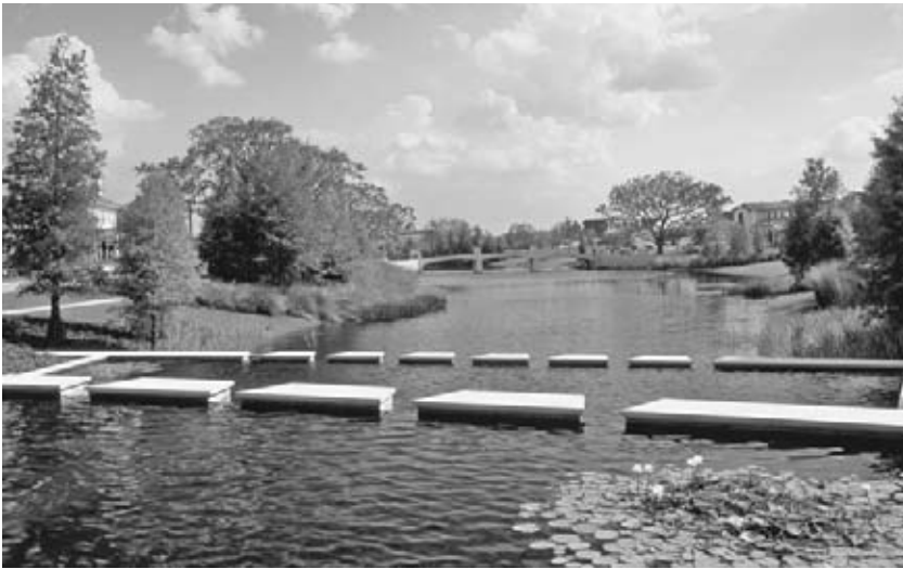
Figure 4.17 At Baldwin Park, Orlando, Florida, a small lake was constructed to manage stormwater. Baldwin Park is a New Urbanism development that emphasizes smart growth principles. Image courtesy EDAAW.
