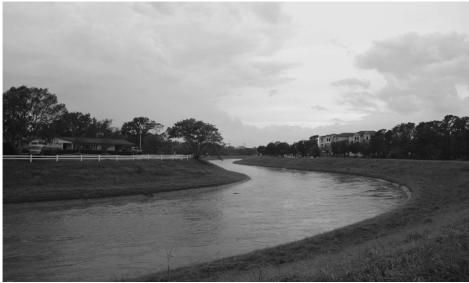
Figure 3.82 The primary purpose of the Brays Bayou Flood Damage Reduction Project is to reduce flooding. Image courtesy U.S. Army Corps of Engineers.
