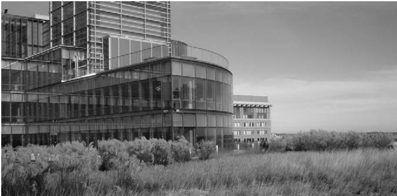
Figure 3.18 The headquarters for the American Society of Landscape Architecture, which is located in Washington, DC, features a green roof. The society is monitoring the roof to determine successes and challenges. Image courtesy ASLA.
