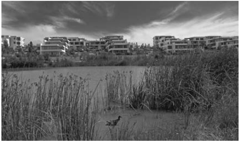
Figure 3.27 The housing units in the Olympic Village stair-step down the hill to take advantage of natural ventilation and southern exposure and to offer views of the wetlands and nature preserve. Image courtesy EDAW.
