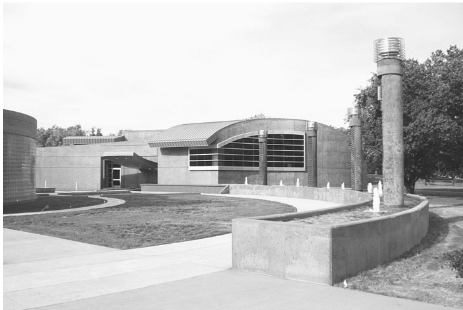
Figure 4.70 The Wichita Area Treatment, Education, and Remediation (WATER) Center serves as both a treatment system and an environmental education center. Image courtesy city of Wichita.
