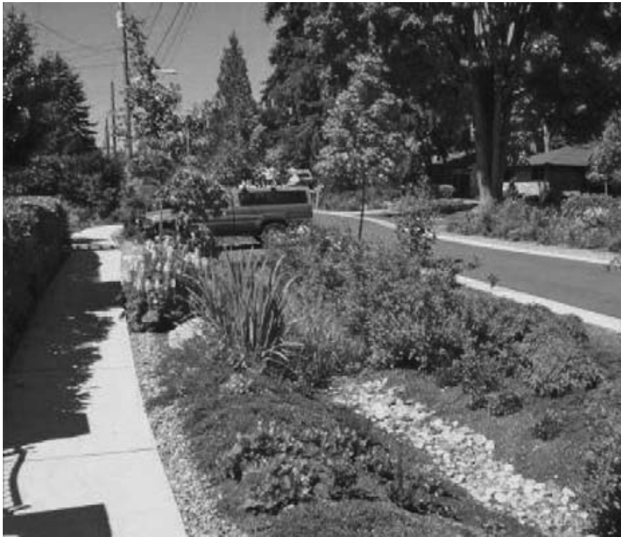
Figure 2.18 In Escondido, California, bioswales are being used to capture stormwater runoff. Bioswales keep the stormwater from running into storm pipes, and this helps reduce the demand on stormwater infrastructure. Image courtesy EDAW.
