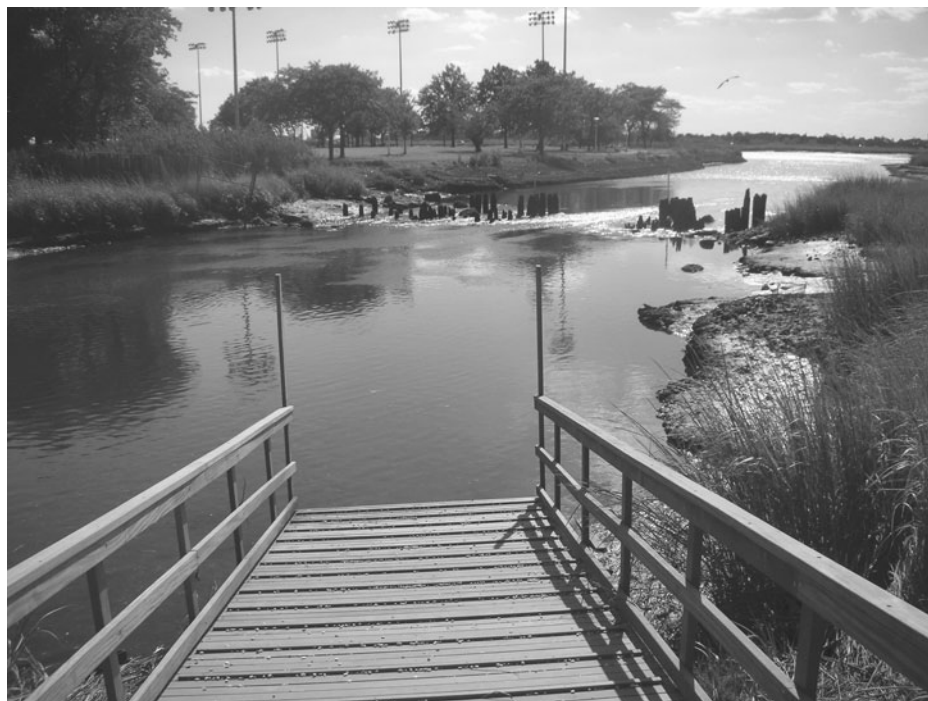
Figure 4.105 Idlewild Park helps manage stormwater runoff from the JFK International Airport. Image courtesy EDAW.
