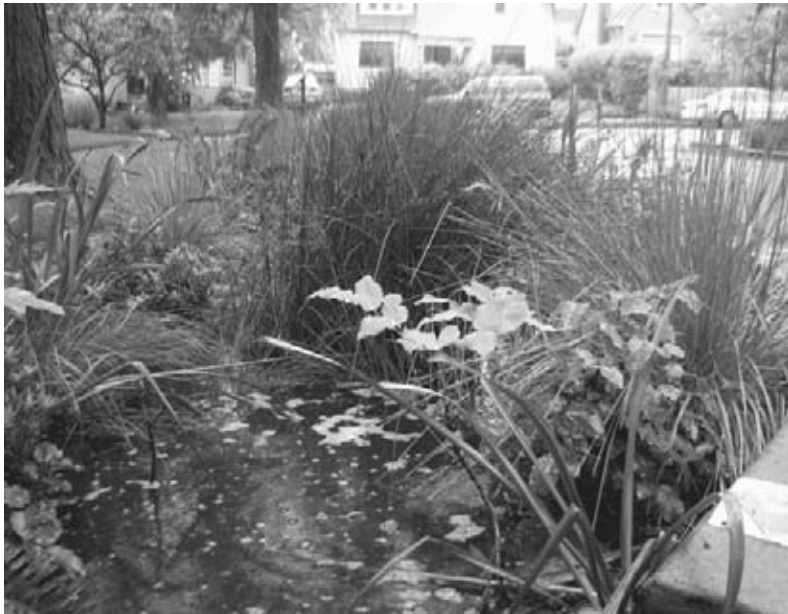
Figure 4.63 The planters can hold up to 85% of the rainwater from a 25-year storm. Image courtesy City of Portland.
