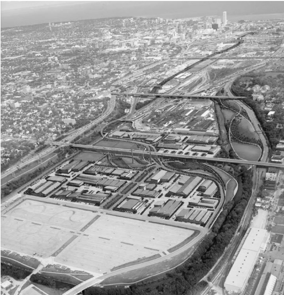
Figure 3.67 The Menomonee Valley Community Park is intended to manage storm runoff for a neighboring light industrial development. Image courtesy Wenk Associates.
