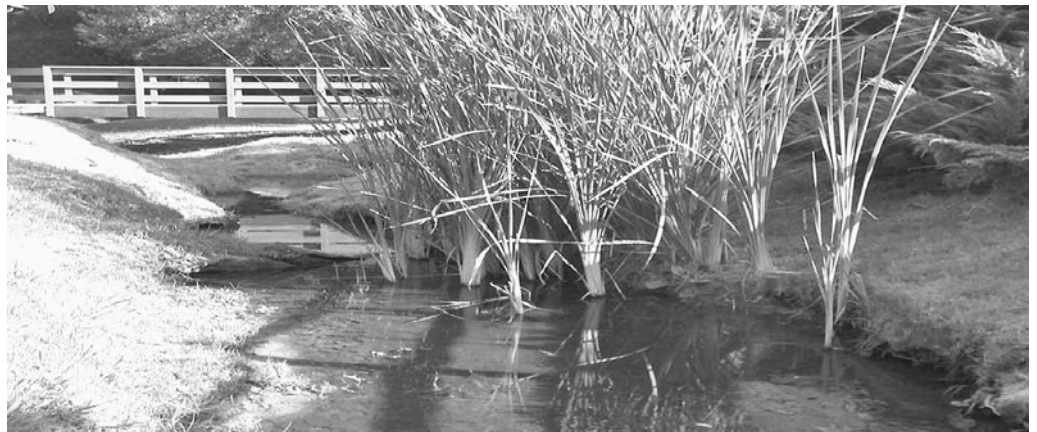
Figure 4.44 Deep-rooted plants were used to help stabilize this streambed in San Diego, California. Image courtesy EDAW.
