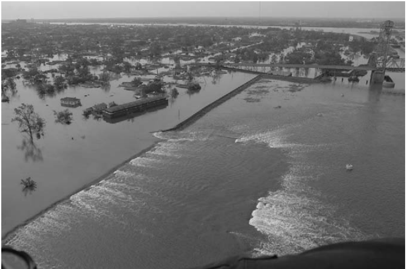
Figure 1.12 When Hurricane Katrina hit the Gulf Coast in 2005, it devastated much of New Orleans. Stormwaters that breached a levee flooded most of the Ninth Ward. Image courtesy FEMA.
