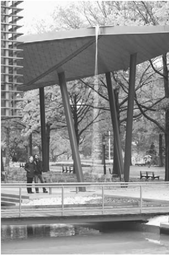
Figure 4.85 Water is an integral part of the site. Rainwater from the roof cascades down into a shallow pool. Image courtesy BSKS Architects.
