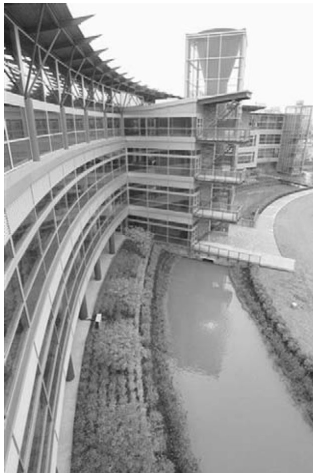
Figure 4.90 The Heifer International Headquarters is located on the site of a reclaimed brownfield. Image courtesy Heifer International.
