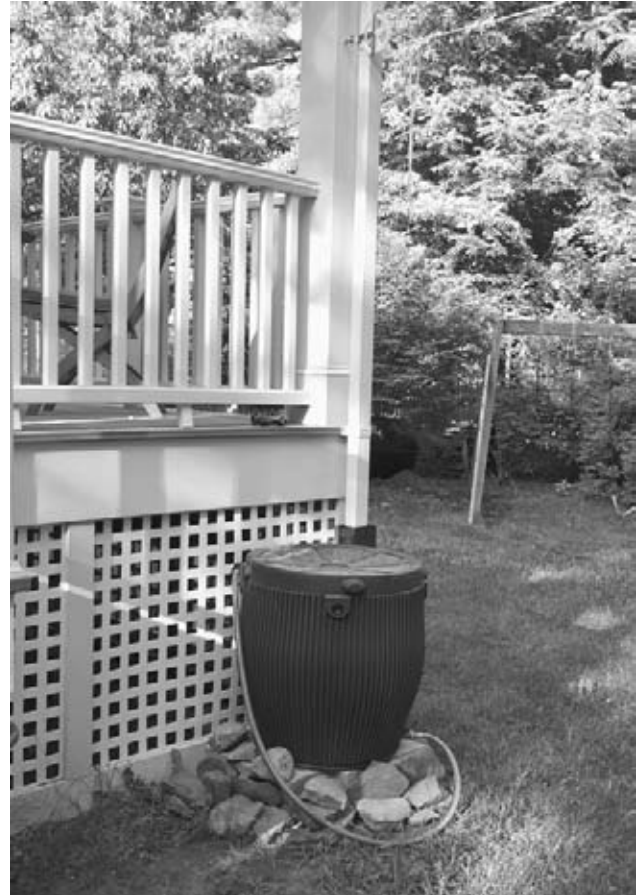
Figure 4.46 Rain barrels can be used to help harvest rainwater at individual houses. Image courtesy NRCS.
