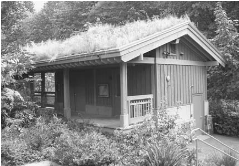
Figure 4.80 Green roofs are used on the smaller structures at the center. Image courtesy Seattle Public Utilities.
