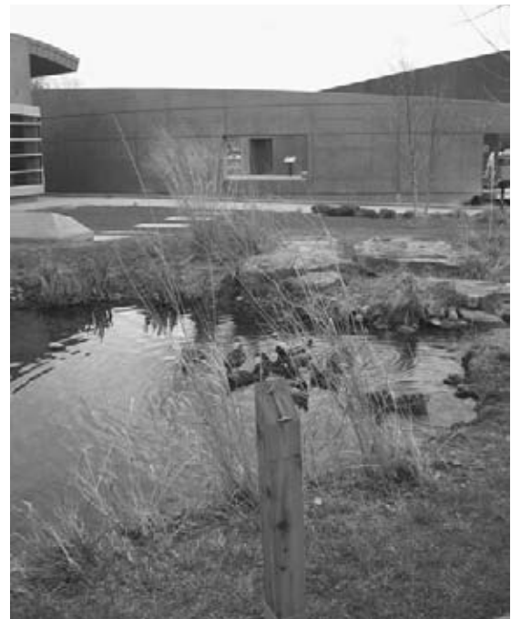
Figure 4.72 Treated groundwater is used on-site for both formal fountains and natural pools such as these. Image courtesy city of Wichita.
