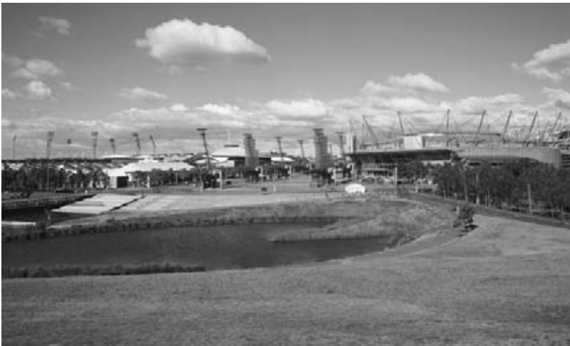
Figure 3.26 Constructed wetlands are used to capture and filter stormwater runoff from the Olympic Park. Image courtesy EDAW.
