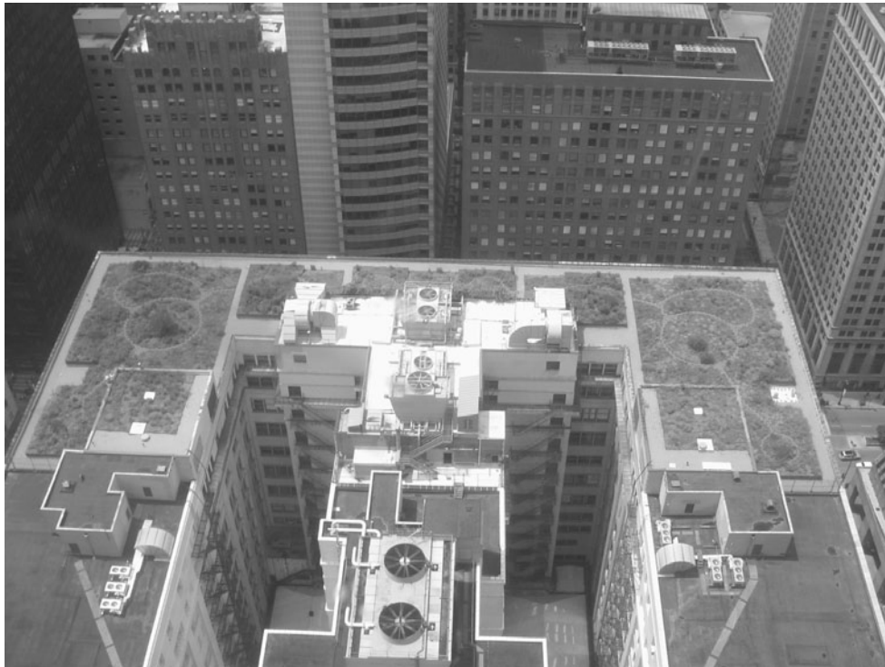
Figure 4.102 The Rooftop garden at Chicago's City Hall building was installed in an effort to improve air quality, conserve energy, and reduce stormwater runoff. Image courtesy city of Chicago.
