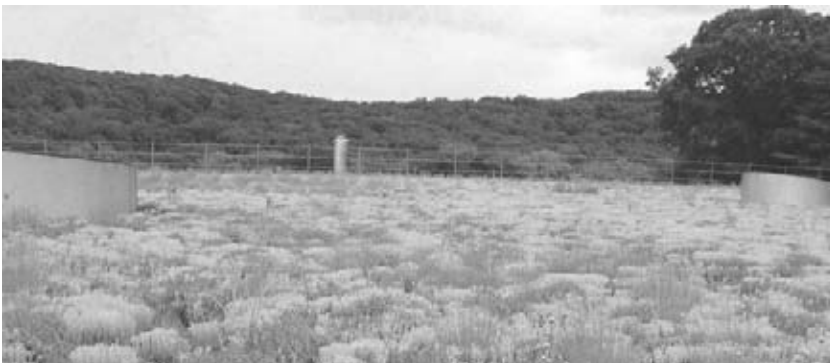
Figure 4.96 The green roof helps create a parklike setting for the treatment facility. Image courtesy Regional Water Authority.
