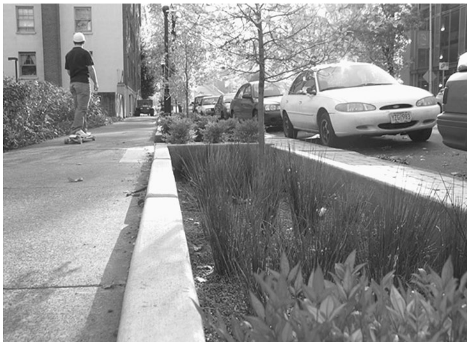
Figure 4.59 The SW 12th Avenue Green Street Project captures stormwater and redirects it into a series of planters. Image courtesy City of Portland.
