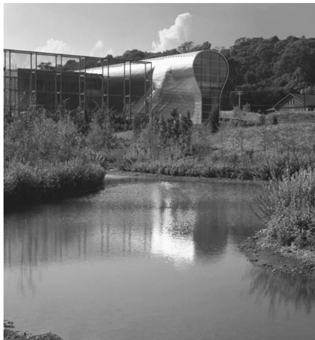
Figure 4.97 The pond on site is used for stormwater detention. Image courtesy Regional Water Authority.
