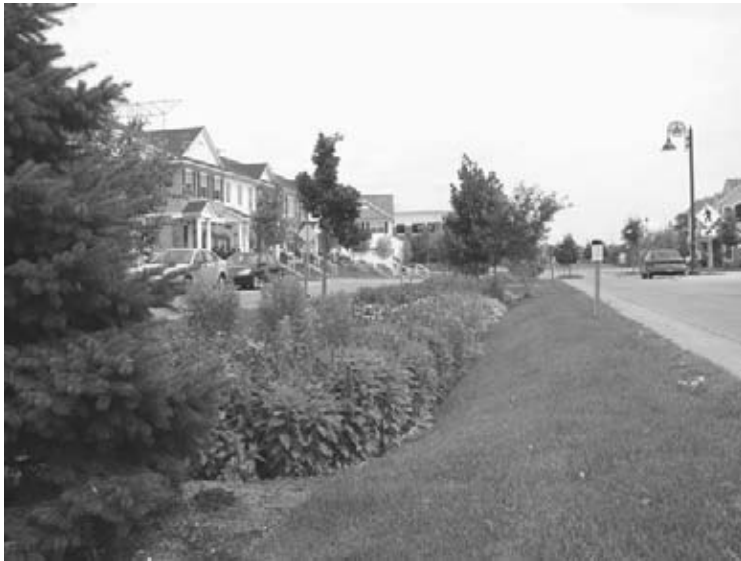
Figure 4.98 One example of how rain gardens are being integrated into site design is the Legacy Village Development, a townhouse development set on 20 acres. Image courtesy Jamie Csizmadia.
