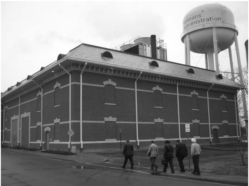
1-6. Cogeneration Facility Using Landfill Gas in Johnson City, TN
