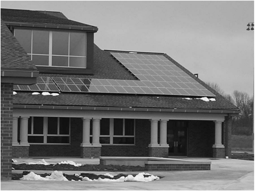
4-7. Solar Collector Array at Twenhofel Middle School, KY
