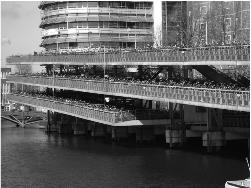
11-2. High-Rise Bike Garage at Amsterdam Railway Station (photo—Mike Clust)
