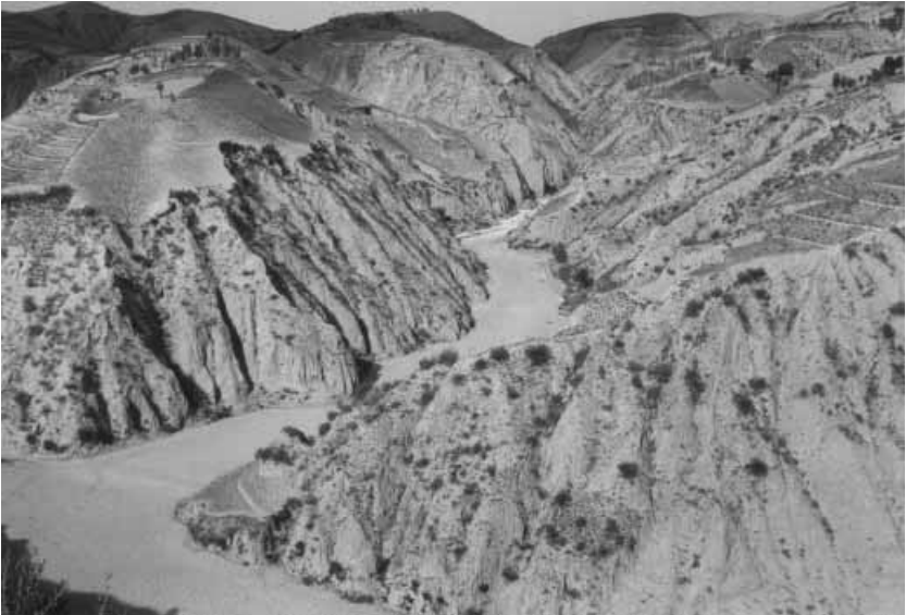
Figure 1.4. This severely degraded landscape in Shaanxi Province, People's Republic of China, is relatively nonfunctional, since it is unable to capture or retain soil, nutrients, water, or organic materials flowing through the landscape. The silted-in reservoir illustrates the magnitude of erosion problems on this landscape. Since little water moves into the soil and there is little vegetation to moderate environmental extremes, it is difficult for plants to become established. Recovery of this site will require physical modifications that reduce abiotic limitations imposed by the lack of vegetation. Despite steep slopes, this area has the ecological potential to develop into forests that stabilize the landscape and retain a high percentage of resource flows. However, socioeconomic pressures (high human population) greatly restrict that option on this landscape.
