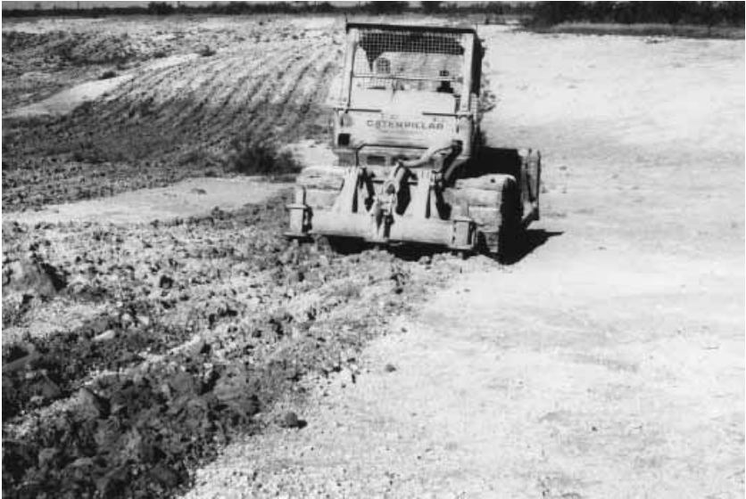
Figure 6.2. Deep ripping (0.4–0.6 m) this highly compacted substrate in west Texas was necessary before water would move into the soil. Ripping or deep plowing was necessary to get any establishment of planted species in this seedbed.
