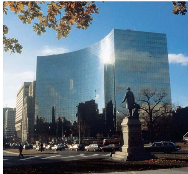
(b) A superinsulated office building in Toronto, Canada, has south-facing windows with insulating glass. The building is so well insulated it uses no furnace. (Courtesy Ontario Hydro)
