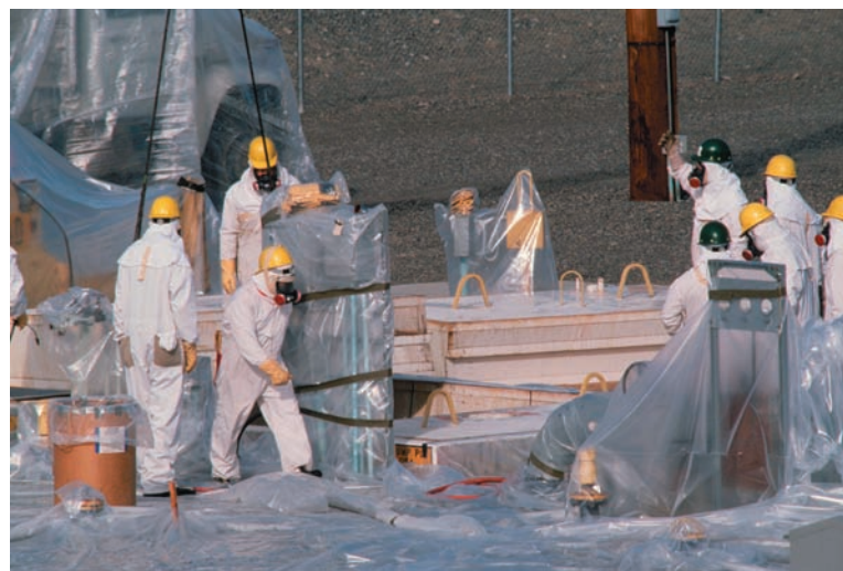
(b) Workers wear protective clothing and respirators to pump 1 million gallons of high-level radioactive waste at Hanford. (Roger Ressmeyer/©Corbis)
