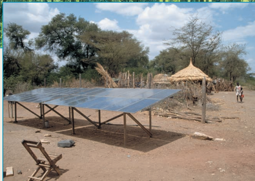
Array of solar panels in rural Kenya. The panels shown here convert solar energy into electricity, which can then be stored in a battery and used to run lights and small appliances. (Liba Taylor/©Corbis)
