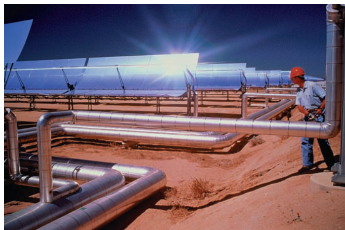
(a) A solar thermal plant in California uses troughs to focus sunlight on a fluid-filled tube. (L. Lefkowitz/Taxi/Getty Images)
