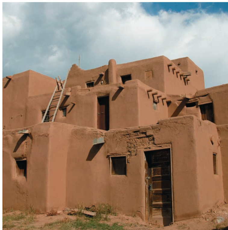
Figure 13.2 Adobe home in the southwestern United States. Adobe has been used for centuries in the southwestern United States, and similar materials can be found in hot, arid regions around the world. Thick walls and carefully placed windows allow the temperature of the building's interior to remain relatively stable through the day and across the seasons. (Altrendo Images/Getty Images)
