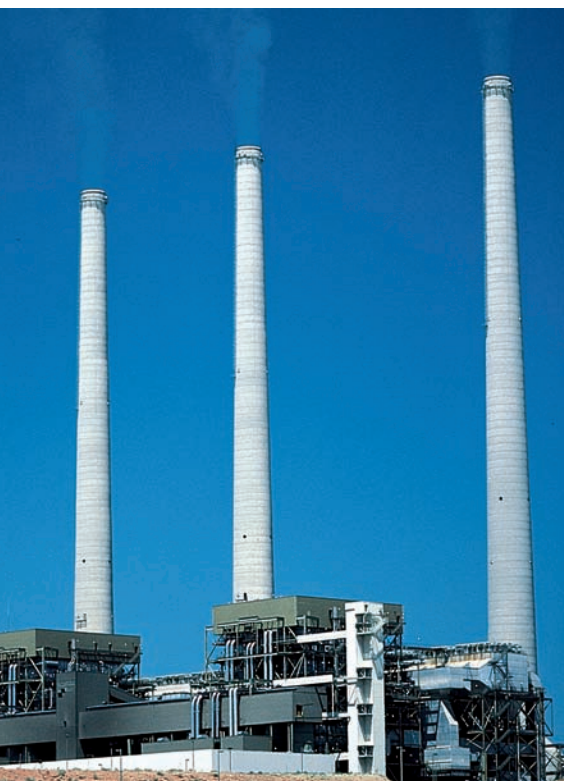
Figure 2.8 Tall smokestacks. Such smokestacks, which emit sulfur dioxide from coal-burning power plants, were exempt from the requirement of pollution-control devices under the Clean Air Act of 1977. (Albert Copley/Visuals Unlimited)
