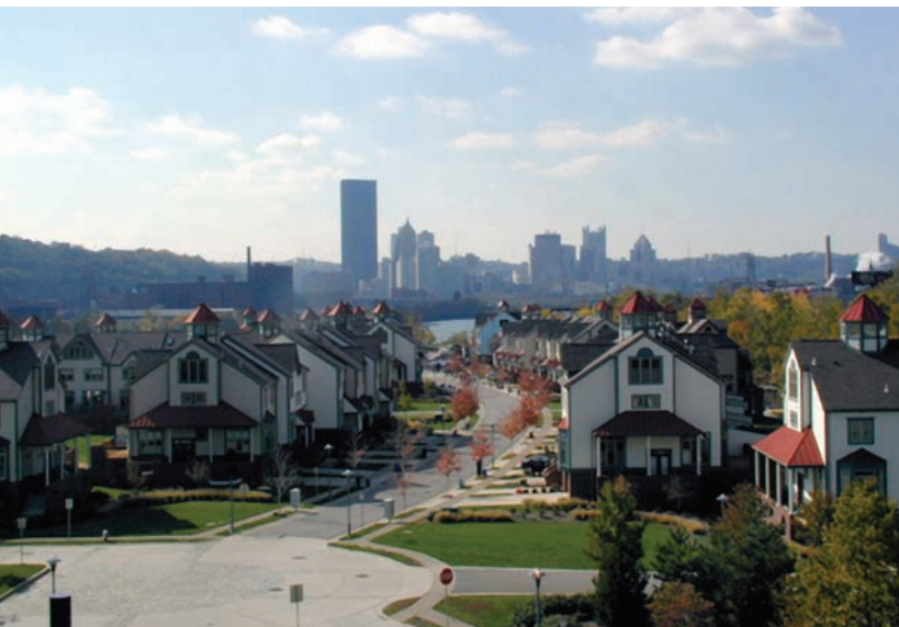
Figure 10.8 Brownfield redevelopment in Pittsburgh. Pittsburgh's first brownfield redevelopment project, Washington's Landing at Herr's Island, today features upscale housing, recreation, and commerce. (Courtesy of Fourth River Development LLC)
