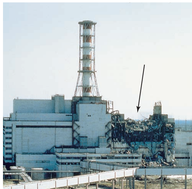
Figure 12.9 Chornobyl. The arrow indicates the site of the explosion. The upper part of the reactor was completely destroyed. (©Novosti)
