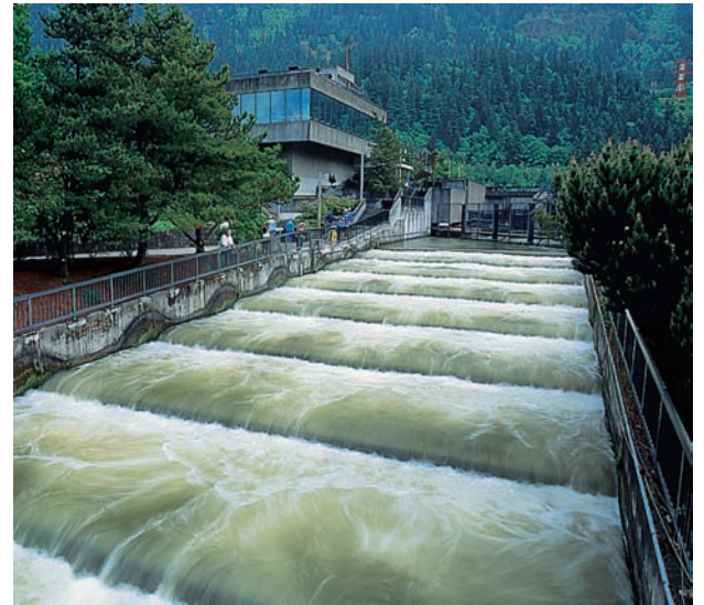
Figure 14.22 Fish ladder. This ladder is located at the Bonneville Dam along the Oregon side of the Columbia River. Fish ladders help migratory fishes to bypass dams in their migration upstream. (©Raymond G. Barnes)
