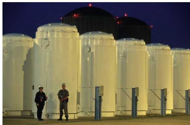
(a) On-site storage casks at the Prairie Island nuclear power plant in Minnesota. Each cask holds 40 spent fuel assemblies (17.6 tons). (Peter Essick/Aurora Photos)
