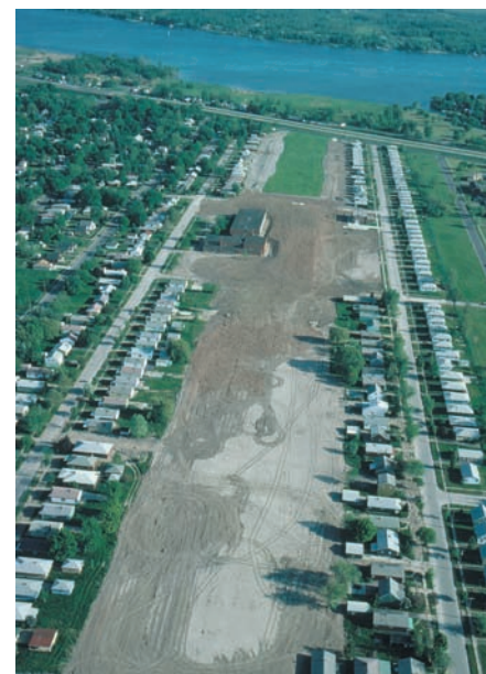
Figure 24.11 Aerial view of Love Canal toxic waste site in the early 1980s. All the homes shown in this photograph were evacuated and demolished. (Andy Levin/Photo Researchers, Inc.)
