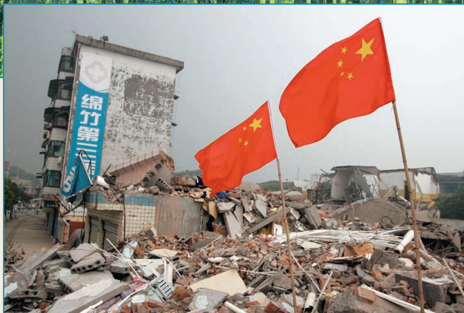
The 2008 earthquake disaster in Hanwang, Sichuan Province, China. The buildings in the foreground collapsed, and the building in the background, although still standing, is unsafe for human occupancy. (Michael Reynolds/epa/©Corbis)
