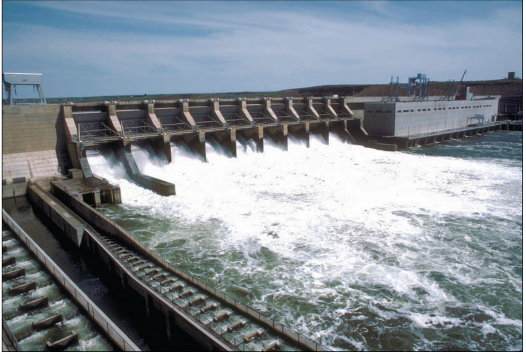
Ice Harbor Dam near Burbank, Washington. Hydroelectric power is a clean, renewable source of energy and generates about 10 percent of the energy in the United States. ( U.S. Army Corps of Engineers, DOE/NREL )
