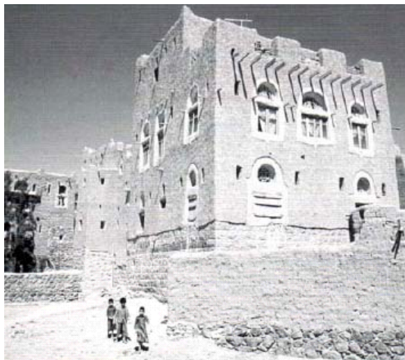
Figure 2: Private house built in the town of Amran in Yemen in 1985 ©CRATEere/EAG
