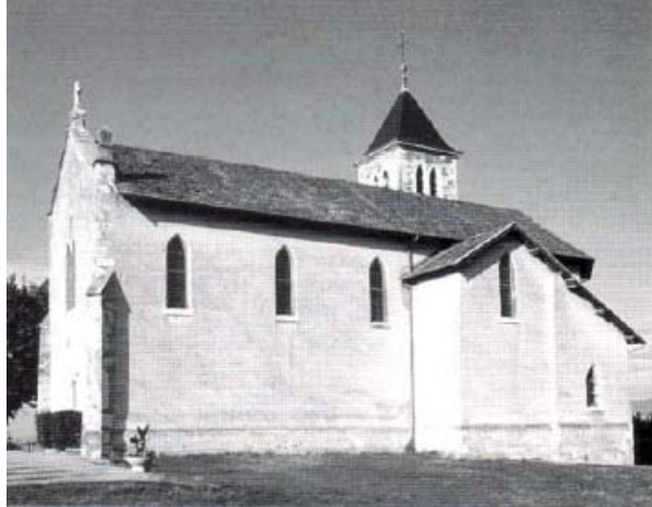
Figure 3: Church built in pisé (rammed earth) at Charancieu in the Dauphiné region of France © CRATerre/EAG
