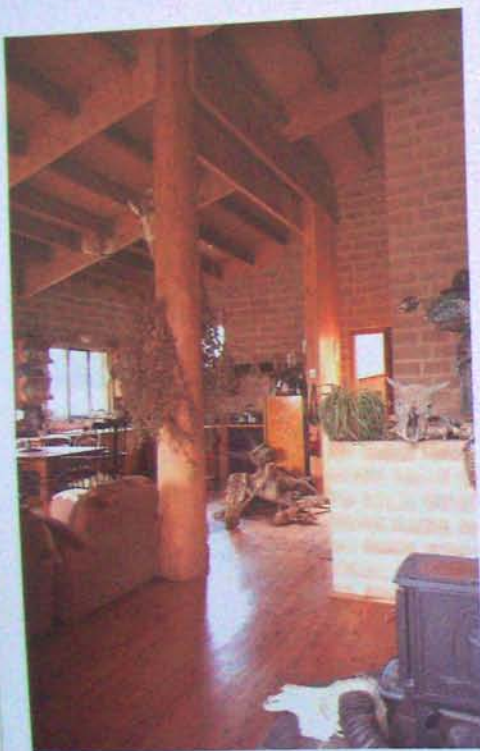
A house with completely natural finishes in the Blue Mountains of NSW, Australia. Elements include Australian recycled pine, compressed earth brick walls, and Australian eucalypt timbers (interior). Planning (architects) Fox-Penner, L. and S. Bayly
