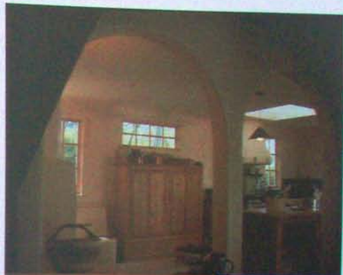
Above: Petaluma residence renovation at Petropopon, California, USA. Floors and worktops are tiled, walls have three coats of natural plaster and a natural-coloured finish. (Architect: C. Venolia; Photograph: C. Venolia)
