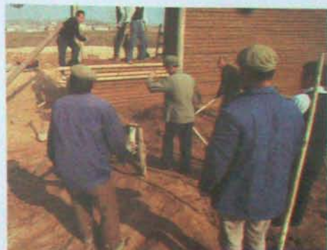
A rammed-earth team in China carry on a tradition thousands of years old
