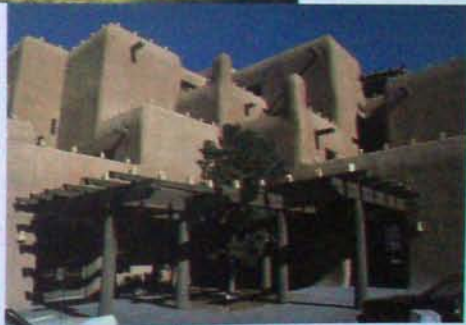
Block construction in Sesto In, New Mexico. Thick earth walls provide excellent sound-attenuation for most frequencies.
