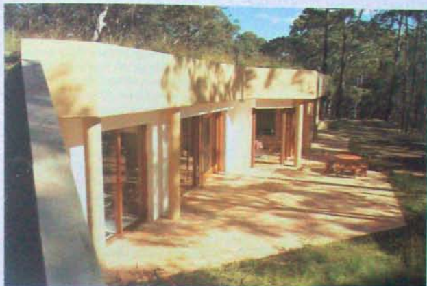
Light-sheltered low-glare house at West Beach, NSW, Australia. Very efficient sound-attenuation by deep earth-cover for all but low-frequency vibration. (Architects: SEA Space Design Pty Ltd)
