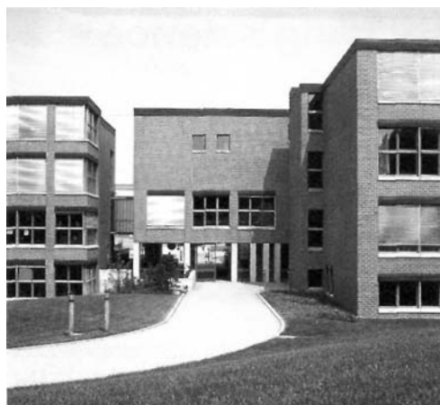
2.5.18 Clay facade elements (Schatz-Preton system)
