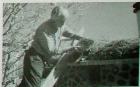
Fig. 8.16: The author installs a moss sod on the edge of the office roof.
