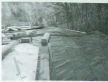
Fig. 8.5 (above): A layer of 6-mil black polyethylene serves as the base of the drainage layer and is installed over the insulation. This is tricky to do on an octagon roof, as the sheet needs to be folded over the saddles between facets, but it is an easy job on a Cove-type roof. We were careful to give plenty of overlap from sheet to sheet (at least 18") and paid attention to the shingle principal when making our overlaps.
