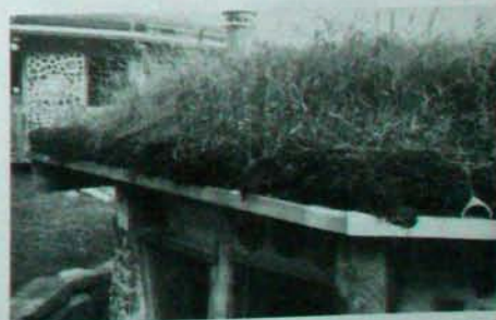
Fig. 8.18: Moss sods drain well, retain the earth and look natural. Note "half-pipe" for drainage.
