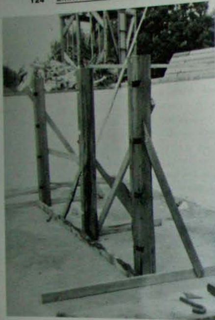
Fig. 6.4: We temporarily braced the support posts for the main girders.
