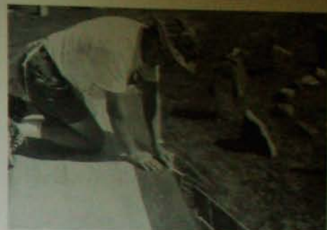
Fig. 7-4: The author bends two inches of the 7" wide flashing over the edge of the 2 x 6" deck.
