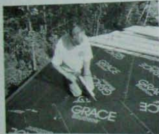
Fig. 8.2 (right): The author caulks the cut edge with Bituthene® Mastic.
