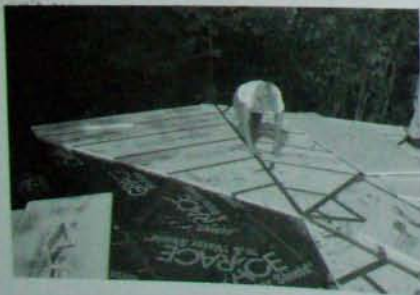
Fig. 8.2 (right): The author caulks the cut edge with Bituthene® Mastic.
