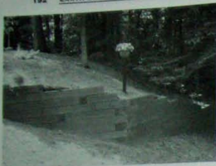
Fig. 9.5: This retaining wall is made of 6 x 6" pressure-treated timbers.
