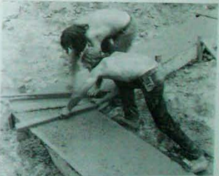
Fig. 3.23: The concrete is screeded with a short, straight-edged board.
