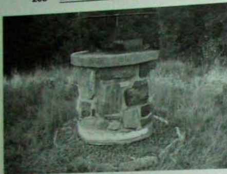
Fig. 11.3: Any projection through the earth roof – skylight, chimney, vent stack – should be surrounded by good drainage material, such as #2 crushed stone.
