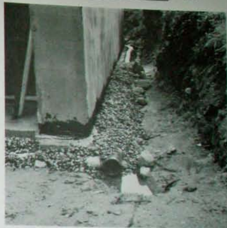
Fig. 7.14: From the lowest point of Log End Cave's footing drain – the southeast corner – the 4" perforated drain tubing continues along the back of the east side retaining wall, finally entering a soakaway.
