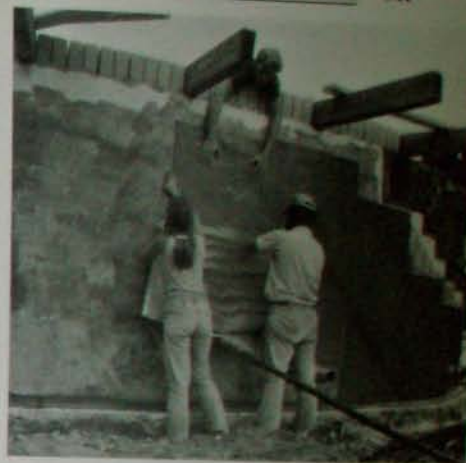
Fig. 7.2: Bituthene® waterproofing membrane is applied vertically to walls.
