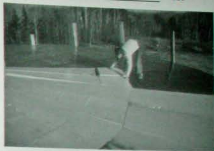
Fig. 7.12: Jaki installs the ship-lapped insulation panels on the Earthwood roof.
