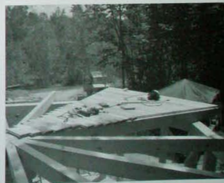
Fig. 6.19: The "waste" from the first cut is used further up the facet, so it isn't waste at all. Next, we would snap chalklines again and trim the two saw-toothed edges.
