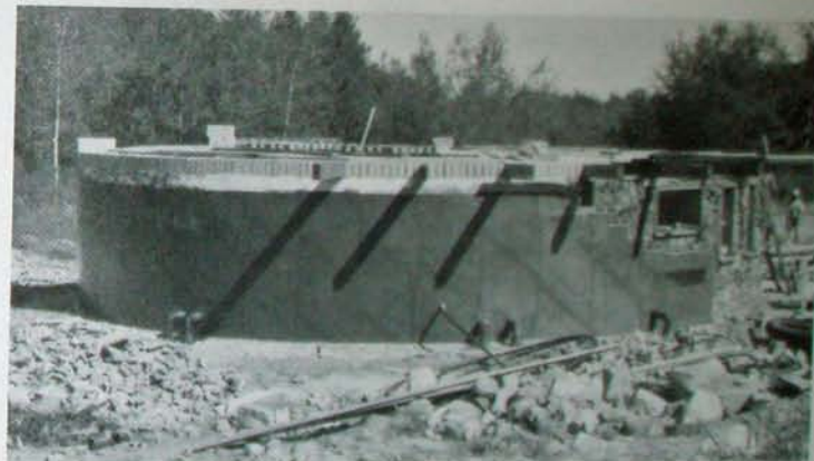
Fig. 7.3: The Bituthene® has been applied to the lower story at Earthwood.
