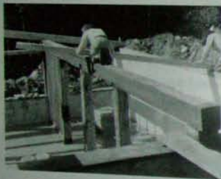
Fig. 6.8: We slide a rafter along the girders.
