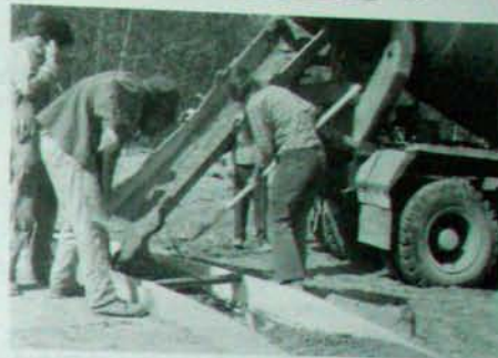
Fig. 3.22: Pouring the footings at Earthwood.
