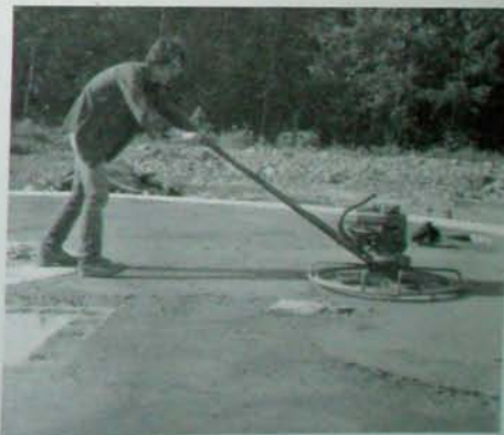
Fig. 4.17: Jonathan Cross power-trowels the slab at Earthwood.
