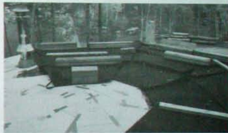
Fig. 8.7 (left): Installing a woodstove chimney. Any projection cut through the membrane has to be treated very carefully, with both waterproofing and drainage. As our Metalbestos® stovepipe has an 8" outside diameter, we made a hole of 12" in diameter through the Bituthene®-covered planking. A reciprocating saw works well for cutting the hole. This way, the chimney has the required 2" clearance from combustible material. The Roof Support Package (Metalbestos® part RSP) unit shown has two adjustable metal flanges which can be screwed to the planking, allowing the installer to plumb the stovepipe itself to a true vertical.
