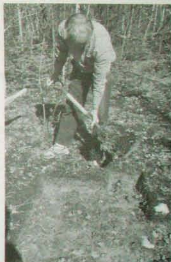
Fig. 8.15: Sodds are cut with a sharp square spade.
