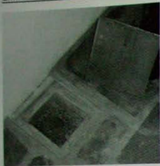
Fig. 4.11: Plumbing cleanout for house drain.
