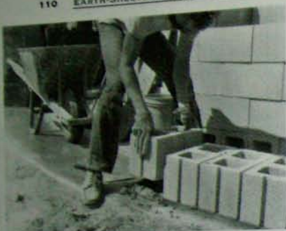
Fig. 5.10: Earthwood: the first course of 8" corner blocks is set in mortar.
