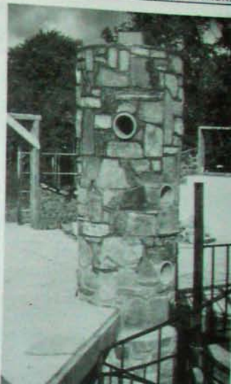
Fig. 10.3: The masonry stove at Earthwood.
