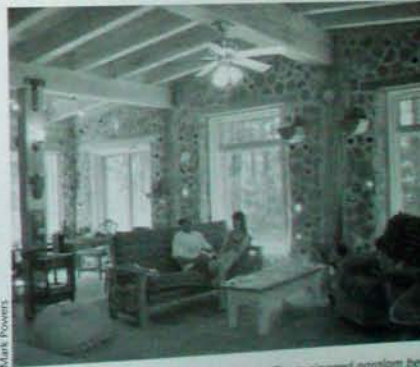
Fig. 12.3: Mark and Mary in their new home. The engineered paralam overhead spans 18 feet.
