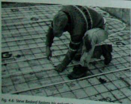
Fig. 4.6: Steve Bedard fastens his polyethylene tubing to the wire mesh with a special rotating hook made for twisting tie bands.
