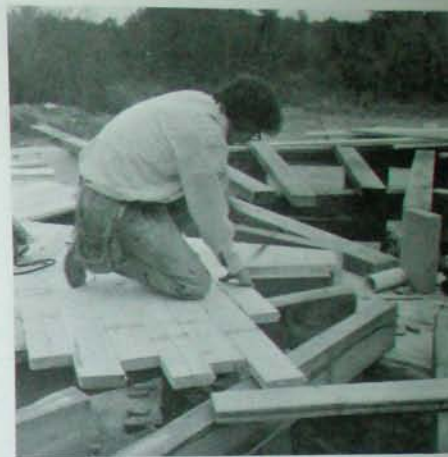
Fig. 6.17: good use is made of short scraps near the center, as seen in Figure 6.17. There are three different situations that arise, which are:
