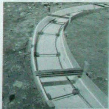
Fig. 3.14: Two-foot by eight-foot sheets of extruded polystyrene, cut as shown at the top and installed as seen at the bottom, fit the footing tracks at Earthwood almost perfectly.
