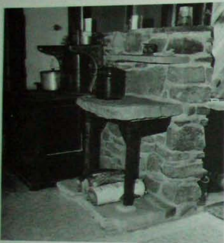
Fig. 10.2: The three-ton room divider at Log End Cave helped the home maintain a steady temperature. background. Use one of the various cordwood mortars described in Cordwood Building: The State of the Art .
