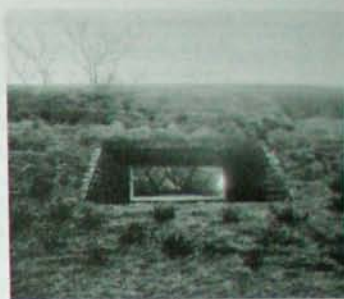
Fig. 1.8 (left): Earthtech 5, a Don Metz design, features a good example of an entranceway penetrating a berm.
