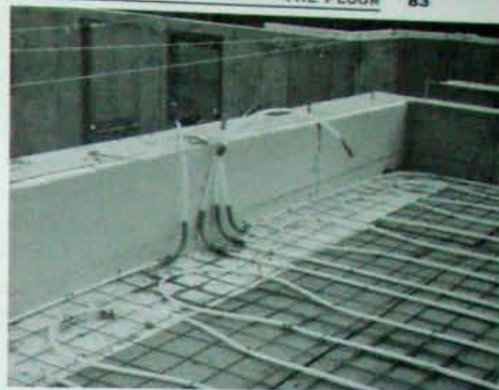
Fig. 4.7: Four different heating zones came together at the edge of the building. At tight 90-degree bends, pieces of rigid plastic fit over the polyethylene tubing to prevent kinking.
