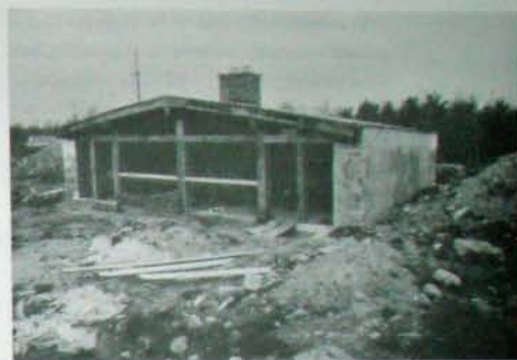
Fig. 2.2: Richard Guay's 40 x 40' Log End Cave, during construction.
