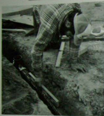
Fig. 4.10: Installation Tips for Underfloor Plumbing Denms Lee checks the slope of the underfloor drains. Plan the plumbing so that all traps are accessible. In the case of a bathtub or shower on the first floor, this will usually necessitate "boxing out" a small area so that concrete cannot get in around the trap or drain. An 18-inch square box made of 2-by-6 material can be seen in Figure 4.9. It provides access to our shower drain and trap. Another good reason for the box is that — thanks to the ubiquitous Mr. Murphy of the famous law — it is very difficult to get the drain in exactly the right place with respect to adjacent walls, which are still non-existent at this point in time. Within the box, you can still make final adjustments to a drain location at the time of shower- or tub-base installation.
