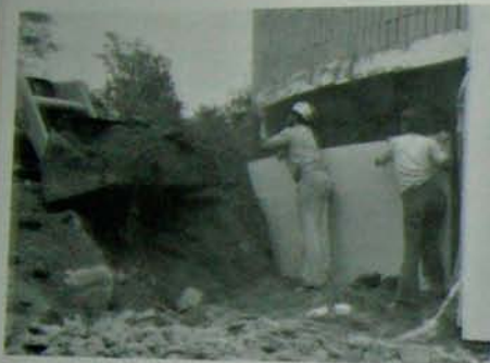
Fig. 7.10: "Bituthene® Protection Board Adhesive" for applying lightweight protection boards, such as extruded polystyrene, to the membrane. Grace warns, however, that the adhesive is extremely flammable and advises installers to read their Material Safety Data Sheet (MSDS), available at < www.graceconstruction.com >, before using it.
