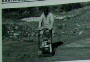
Fig. 3.4: Dennis Lee tamps the sand pad at Earthwood with a power compactor.
