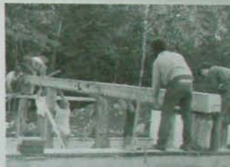
Fig. 6.5: We place the center girder on its posts, Log End Cave.
