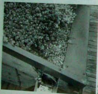
Fig. 8.23: Photograph of the drainage detail at the Dancey home.
