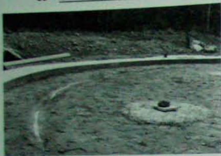
Fig. 4.4: 4" perforated drain tubing is set into the sand pad.
