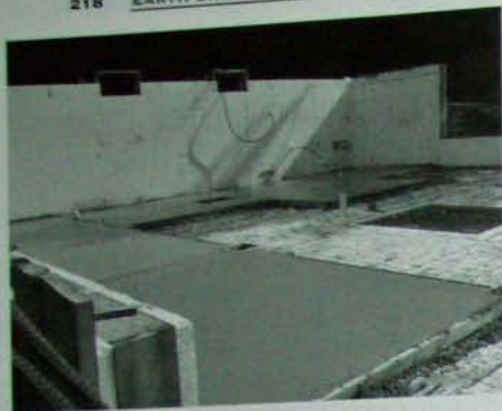
Fig. 12.1: Mark employed a foam-block forming system for his reinforced concrete walls.
