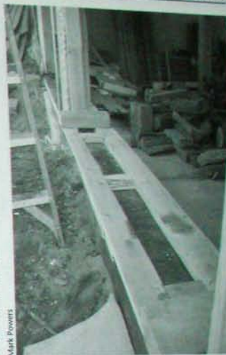
Fig. 12.2: The poured wall is broadened to accommodate the 16-inch cordwood wall by the use of this 2 x 6" detail, described in the text.
