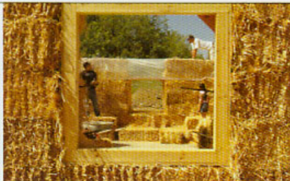
For ease of construction, windows are sized to bale dimensions.
