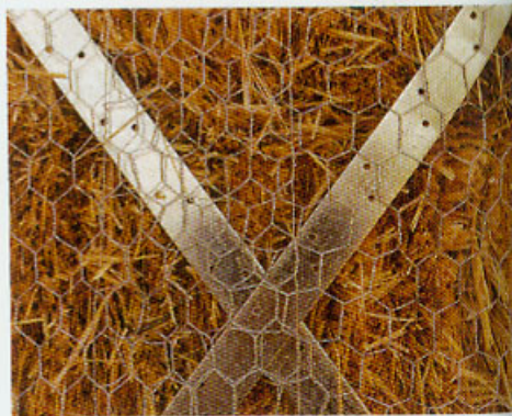
Coil Straps form x-bracing to resist wind and earthquakes.
