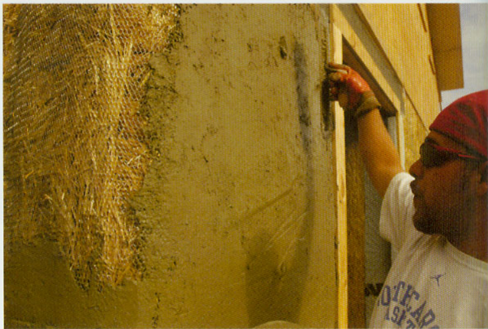
Working the scratch coat toward an exterior corner
