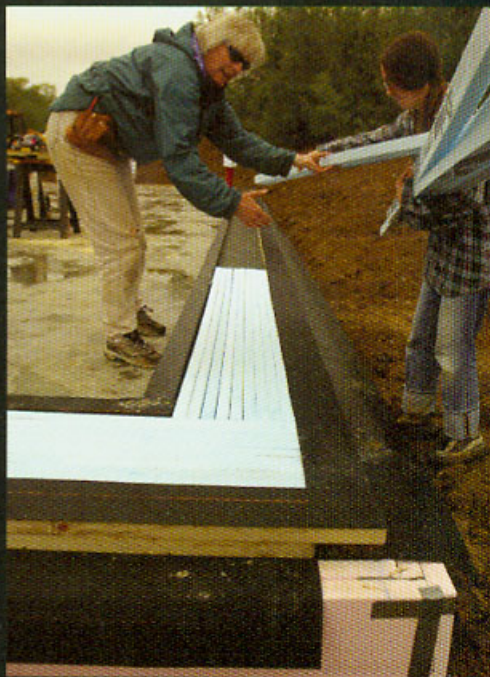
Detail of base plates with insulation
