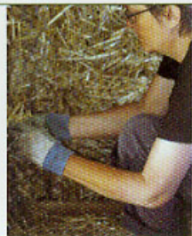
Use loose straw to fill the gaps.
