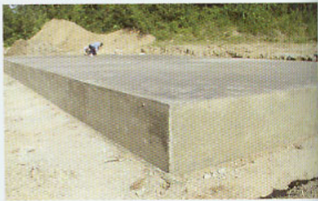
The completed slab awaits straw bales.
