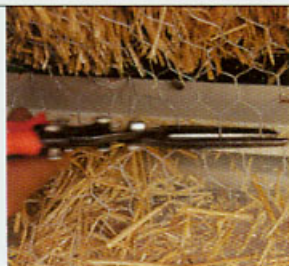
Trimming lath within the weep screed
