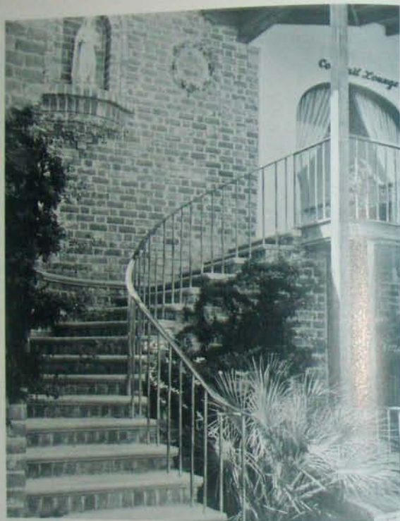
Fig. 3.2 Casas Adobes Shopping Center, Tucson, Arizona. Curving stairway with brick steps and ornamental iron railing provides tremendous charm if the budget permits.
