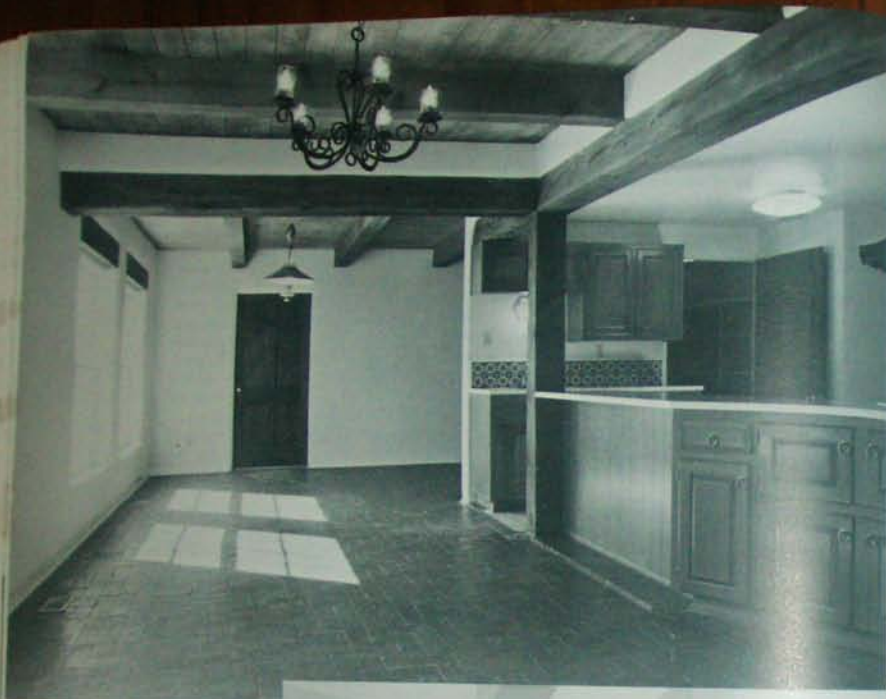
Fig. 7.16 Residence, Albuquerque, New Mexico. Various combinations of lathes may be required to accomplish roof timber framing.
