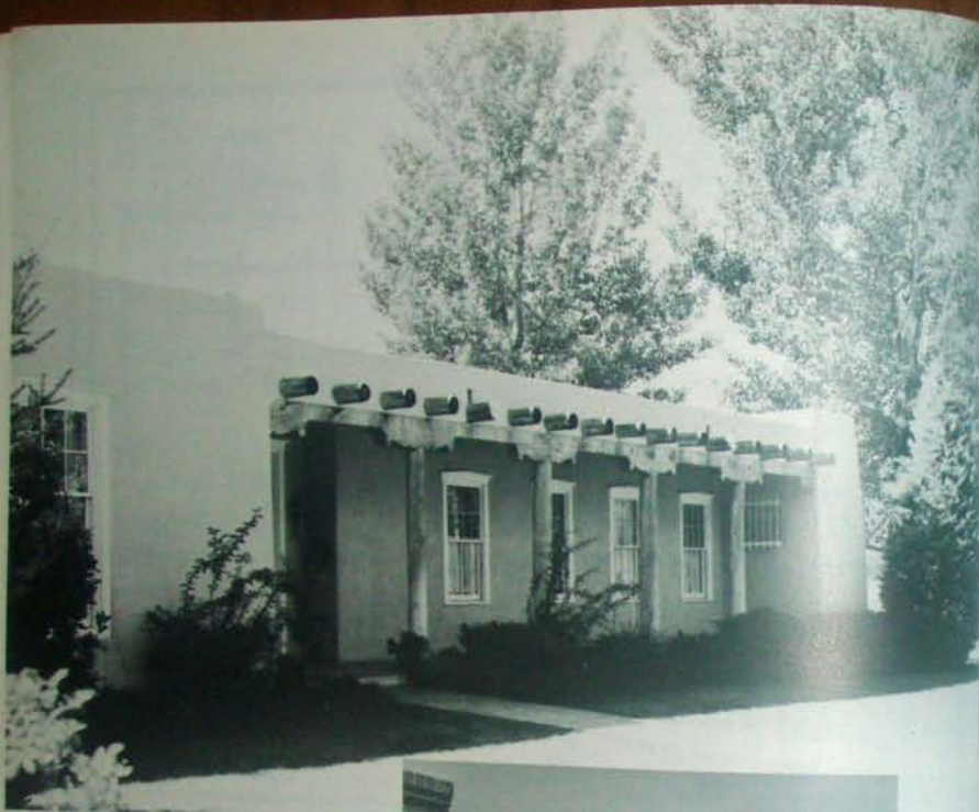
Fig. 2.8 Residence, Albuquerque, New Mexico. An excellent example of the Pueblo style. Note canale (roof drain) concealed in viga .
