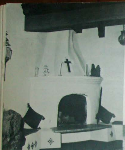
Fig. 18.3 Residence, Albuquerque, New Mexico. P. G. McHenry, Jr., architect-builder. Sculptured plaster for fireplace facing creates an old-world atmosphere. Stone slab for hearth allows for wood storage below.
