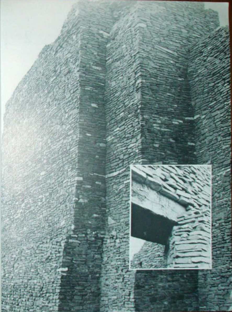
Fig. 1.6 Quarañá Mission, near Montañasire, New Mexico. A Spanish Franciscan mission built in 1625, abandoned in 1670 due to drought and Indian depredations. Multiple corners and thickened lower walls provide strength for this traditional central plan with its extremely high walls. Construction is of interlocking rubble-course and mud mortar. Imagine trying to build this without modern tools and scaffolding. Inset: decorative treatment of squared-beam lintel beam over doorway.
