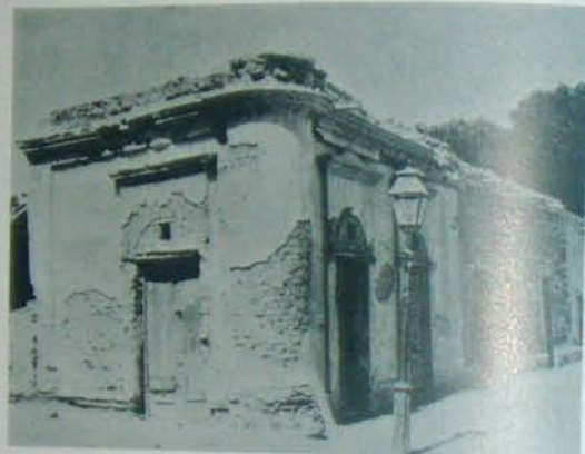
Fig. 2.13 Downtown Tucson, southwest corner of Pennington and Pearl, circa 1883. Note Baroque and Victorian ornamentation done with locally available materials (adobe and plaster). Courtesy Arizona Historical Society.
