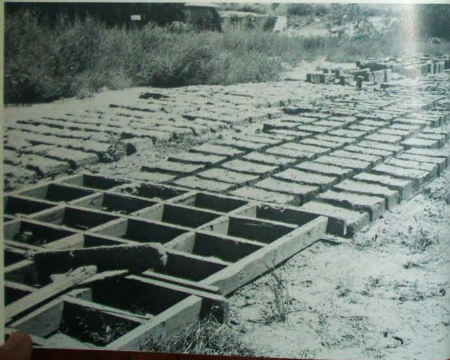
Fig. 7.2 Adobe gang mold. Foreground: Empty molds ready for filling. Center: Damp bricks with mold removed. Background: Bricks turned on edges for drying.
