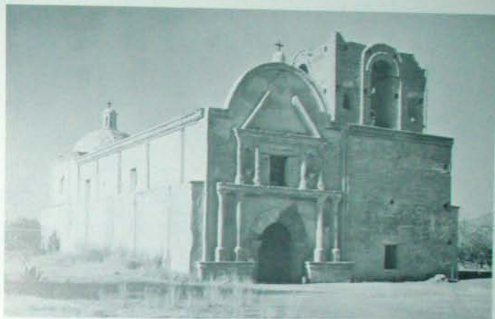
Fig. 2.10 Tumacacori Mission, Arizona, about 1693. Built in the 1790s. Mixture of mud adobe (lower left) and kiln-fired adobes in higher construction at right. Hard-plastered facade provided a good medium for Franciscan style.
