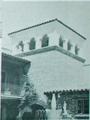
Fig. 2.12 Casas Adobes Shopping Center, Tucson, Arizona. Top: Burnt adobe construction with multiple arch detail. Note that hard-fired brick was used at the arch and support points where the lower compressive strength of burnt adobe might fail. Center: Ornate rafter ornamentation. Bottom: Mission style belltower with ornate arches, mixed materials and styles.
