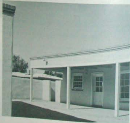
Fig. 2.9 Residence, Albuquerque, New Mexico, P. G. McHenry, Jr., architecture-builder. Modern adobe home detailed in typical Territorial style with coping at wall tops and ornate window and door trim.
