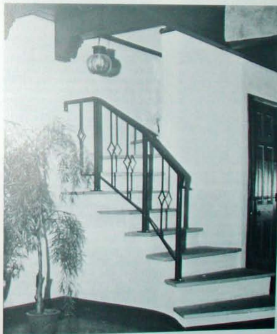
Fig. 3.3 Residence, Albuquerque, New Mexico. P. G. McHenry, Jr., architect-builder. Stairways can be condensed into a small area when necessary. This corner (5' 2") was utilized to provide a stairway to a balcony, with a closet included.
