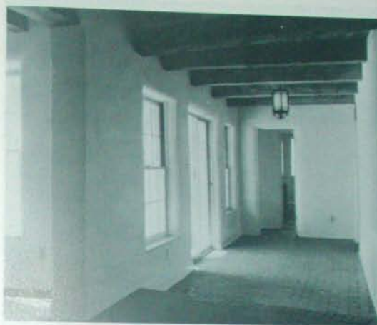
Fig. 3-1 Residence, Albuquerque, New Mexico. P. G. McHenry, Jr., architect-builder. Wide gallery provides a furnishable room in place of a long narrow hall. Change in floor levels may be easily made to fit uneven site (step in foreground).
