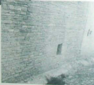
Fig. 1.5 Chaco Canyon National Monument, New Mexico. Progressive improvement in stone building techniques helps date the large number of structures. Notice the bonding course of larger stones at intervals.
