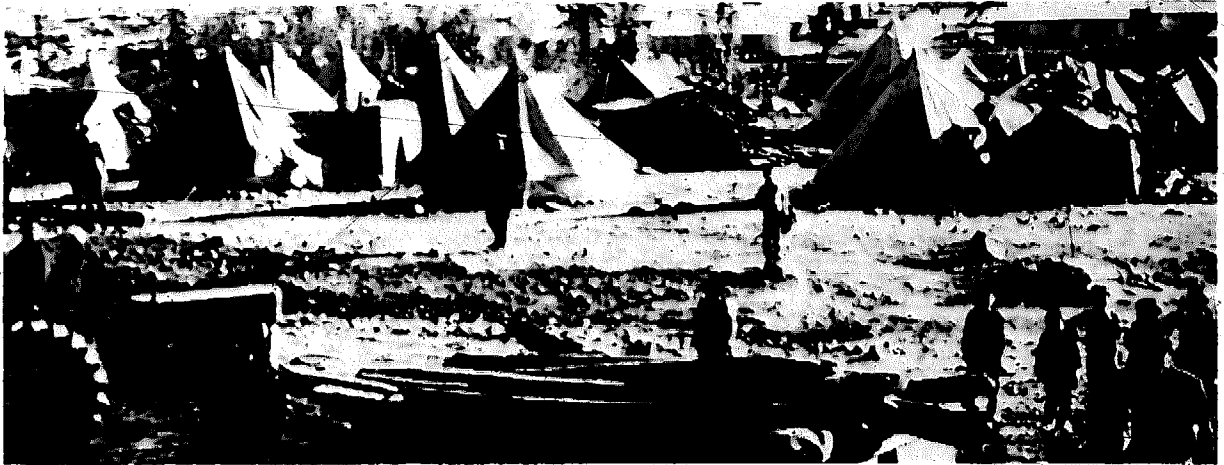
63 Tents provided by Red Crescent in use in Lice, Turkey, eight weeks after the earthquake
