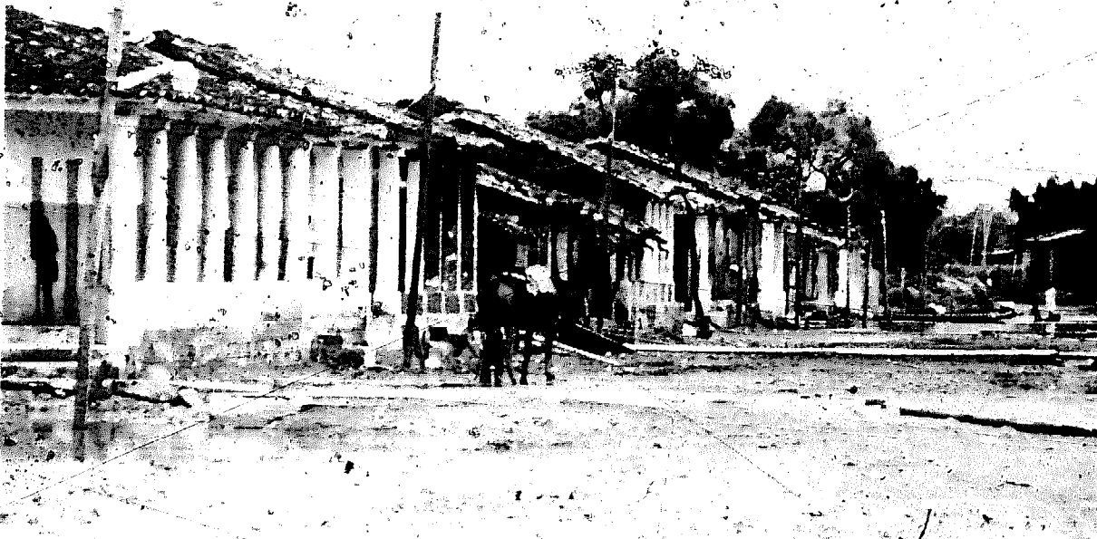
10 Housing in Trinidad, Bolivia, with raised plinths to protect buildings from flooding. In this instance, the flooding was so intensive that its level rose above the elevated floor level.
