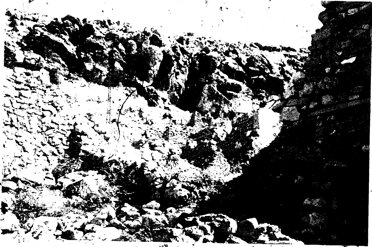
5 Lice, Turkey, following the earthquake of September 1975. Note the vulnerable site below rock formations
