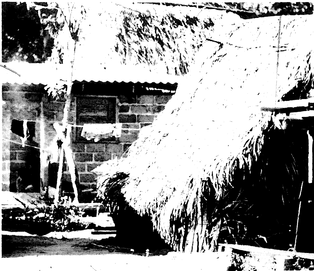
21 The village of La Nueva Jutosa, Honduras, built after Hurricane Fifi, September 1974, showing contrasting forms of new housing – concrete block provided by CARE and traditional thatched homes
