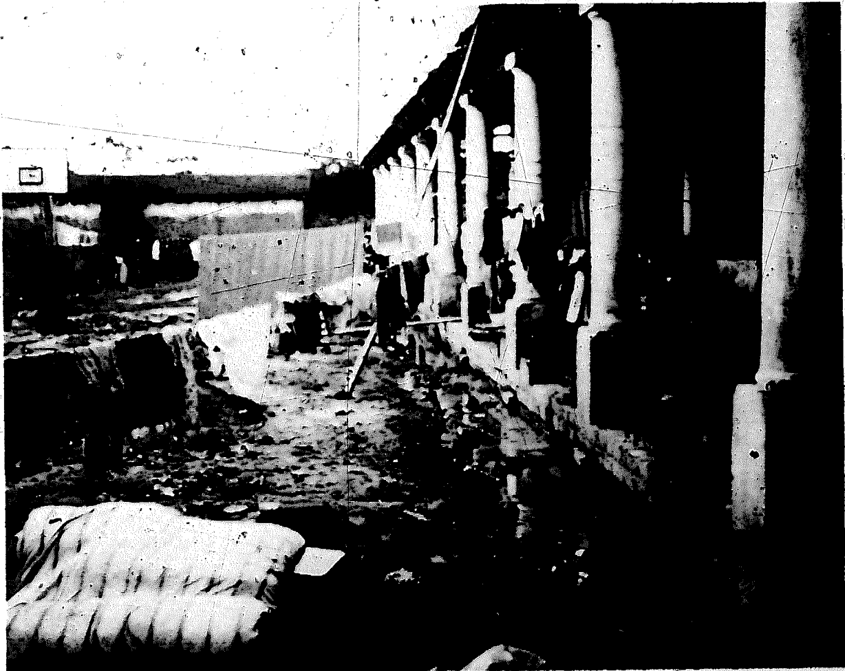
50 Existing buildings form a very valuable resource for housing for homeless families: a converted convent in Trinidad, Bolivia
