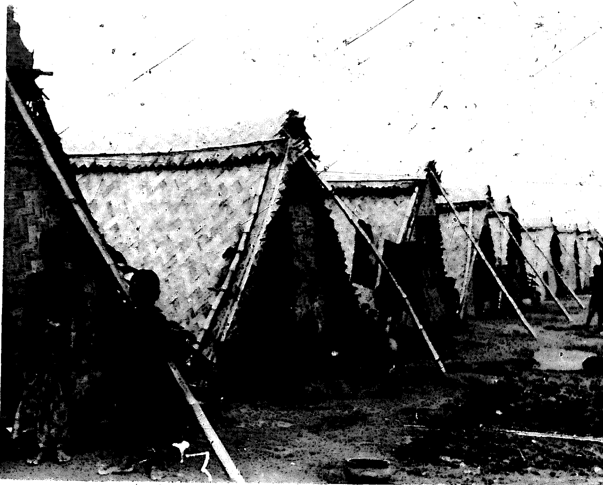
61 Completed 'A' Frame housing at Demra, Bangladesh
