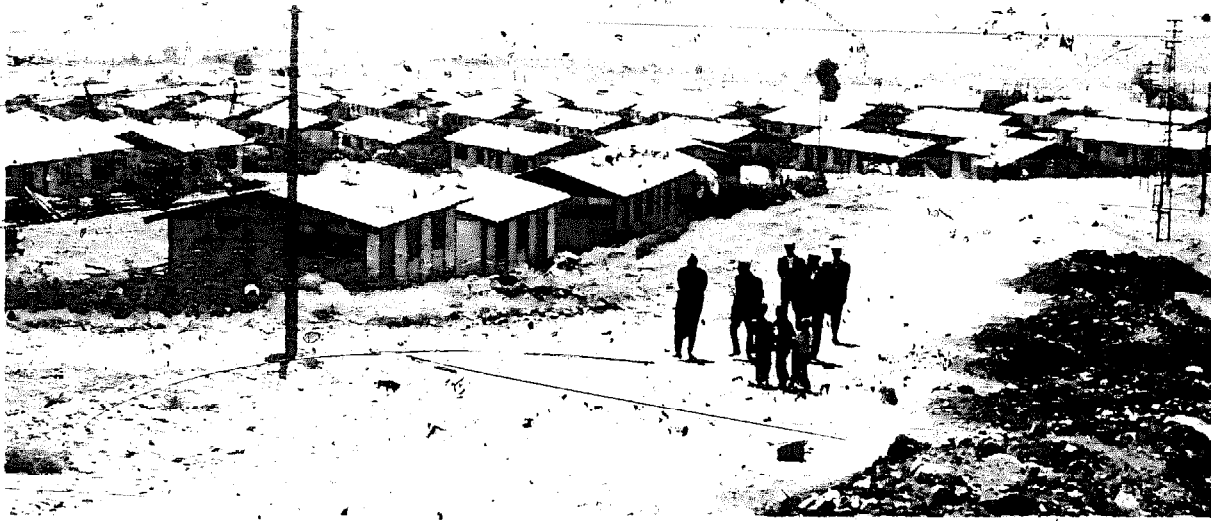
24 Prefabricated houses in Lice, Turkey. 1,500 of these were built within sixty days of the earthquake in September, 1975. (See Ill. 8 for traditional housing)
