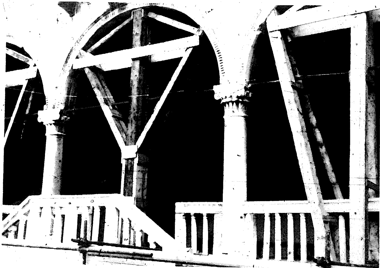
75 A shored-up arch in Gemona, Italy
