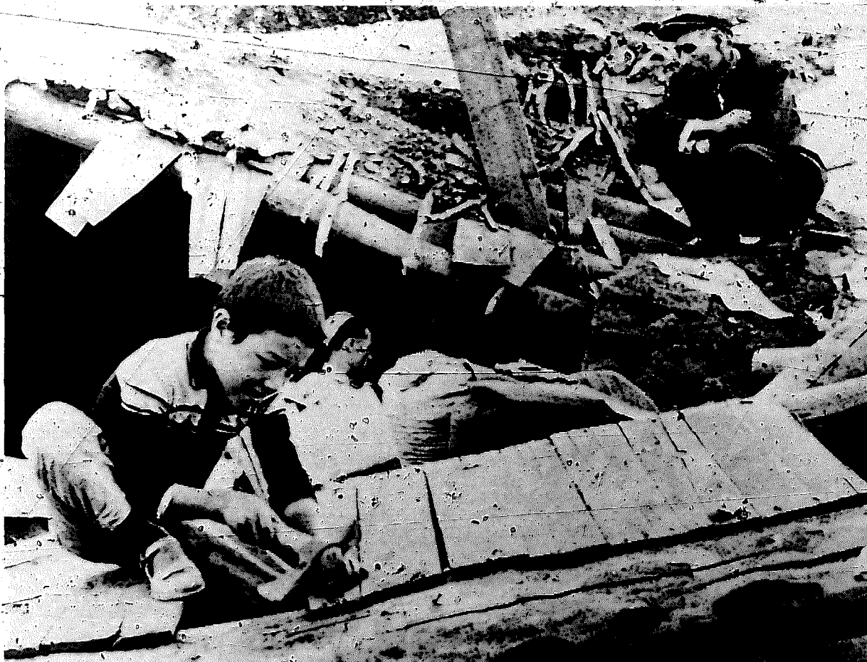
45 A family survey their wrecked home following the Turkish earthquake
