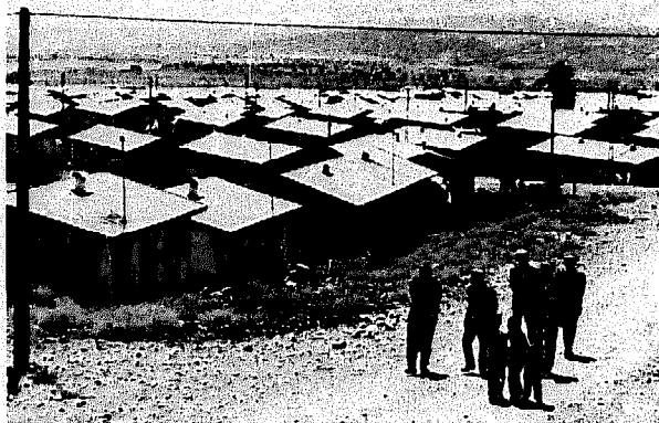
Prefabricated housing built by the Turkish Government at Lice following the earthquake of September 1975. Many families objected to the form and siting of the housing. These objections related to their lack of participation in what was provided, and the cultural and climatic unsuitability of the housing.
