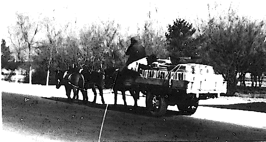
A wooden cart incorporating pneumatic tyres: China.
