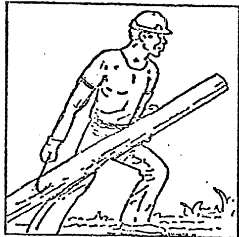
(h) Use two hooks for dragging.
