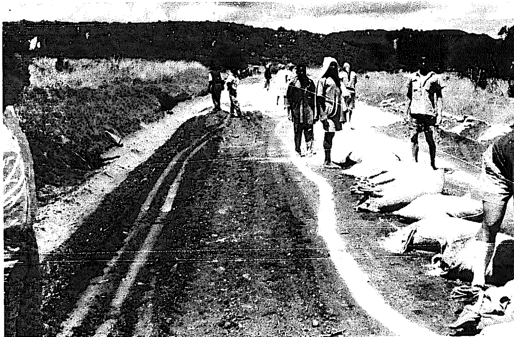
Figure 5. Lime stabilisation: bags of lime are dumped along the road
