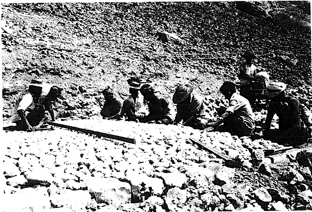
Figure 9. Cobblestone road construction
