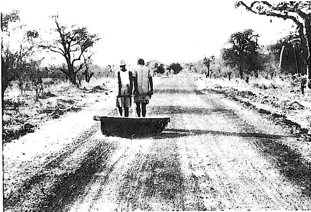
Figure 37. Broom used to finish a road surface (East Africa)
