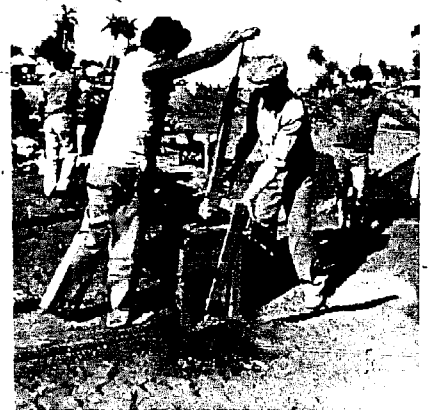
Position of lever just before compaction phase.
