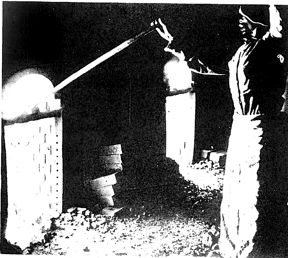
Grates in use in coal fired kiln but excess air can still enter at top and arrangement would not suit woodburning
