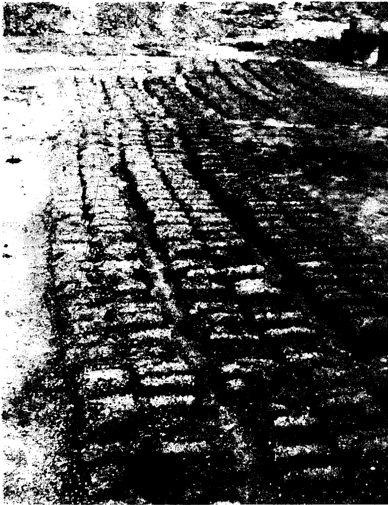
Slop moulded bricks drying in the open destroyed by rain
