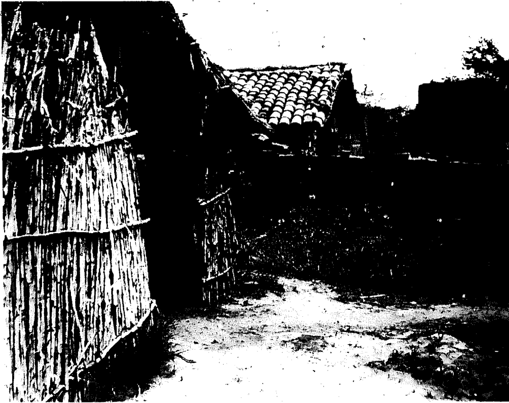
Covered working and drying sheds - building in foreground built in traditional manner of round poles, bamboo and grass
