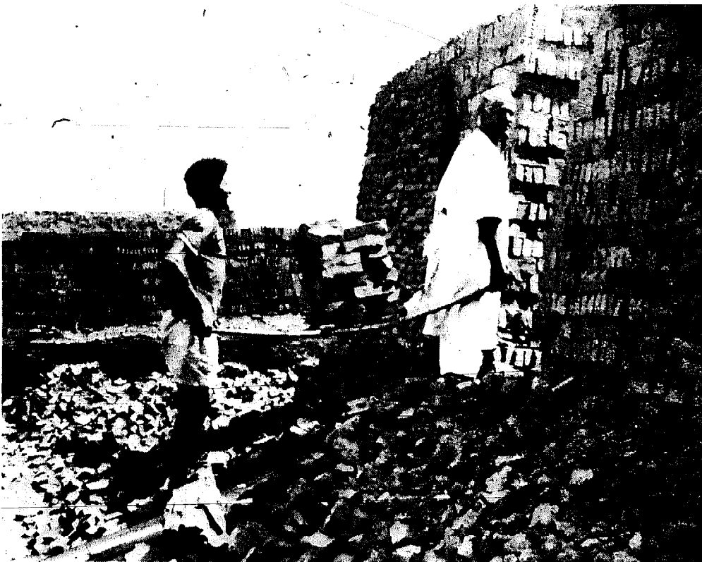
Two men carry dry bricks up to the clamp for setting
