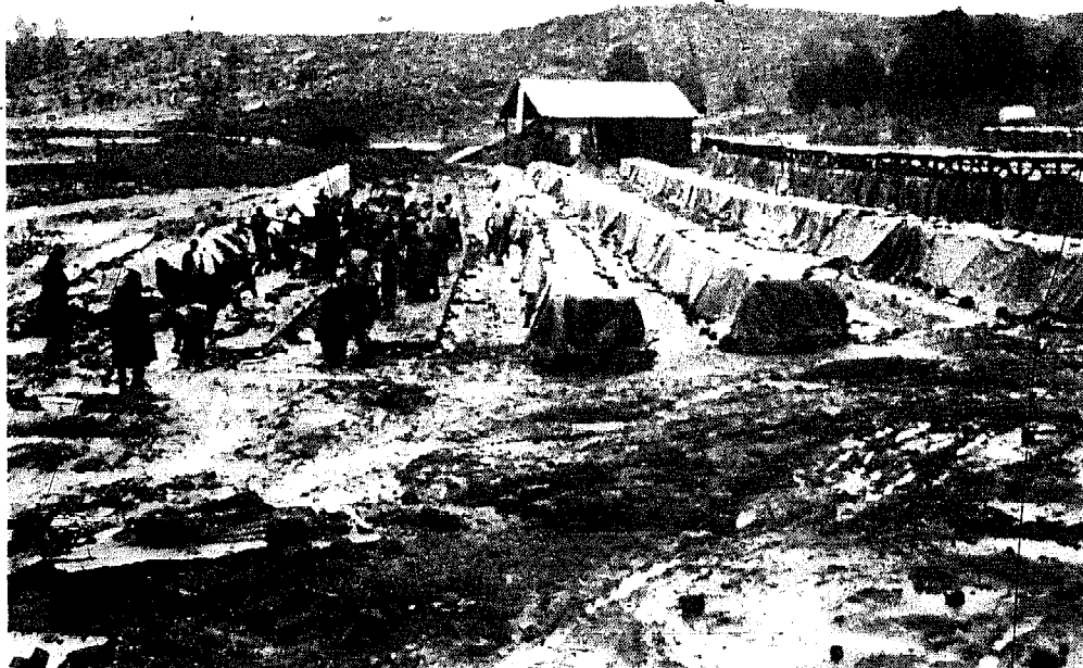
Stack of extruded bricks sheeted over to prevent drying cracks and also as a protection against rain damage. This procedure prolongs the drying period to 3-4 weeks
