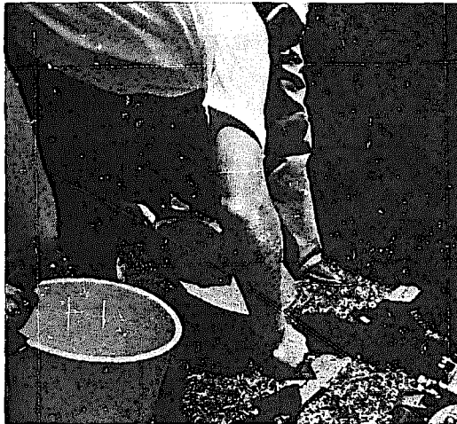
Filling mortar containers .
