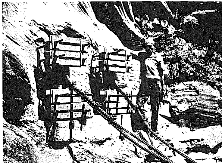
Rock anchors used for main cable anchorage Tatopani (Budhi Gandaki), 1974
