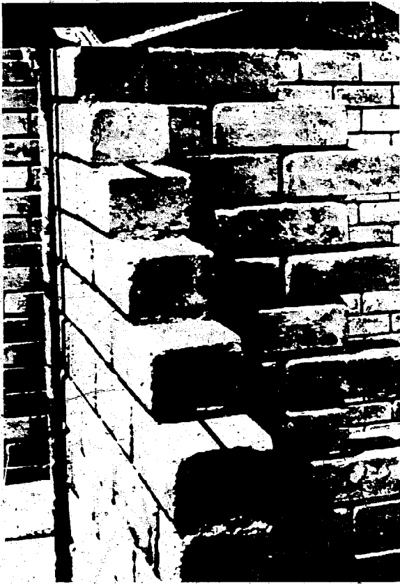
Fig. 66 Extra metal reinforcements for walls of soil-cement blocks are highly desirable in active seismic regions.
