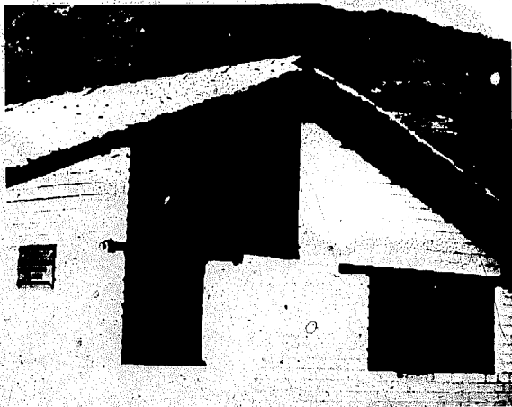
Fig. 73 Wall beam constructed directly onto the wall.
