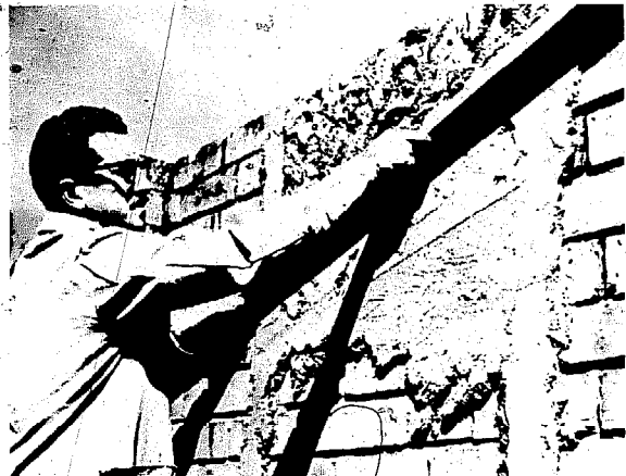
Fig. 91 Using the scraper in plastering a wall.
