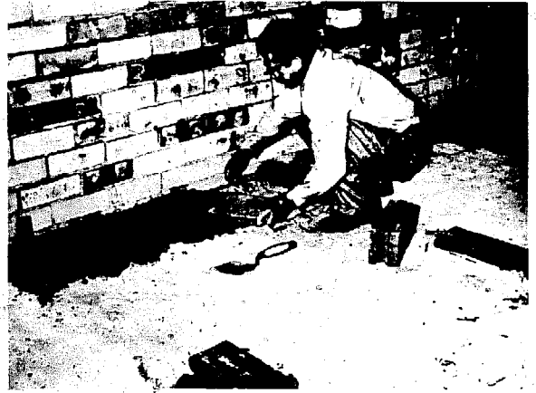
Fig. 86 Laying floor tiles.
