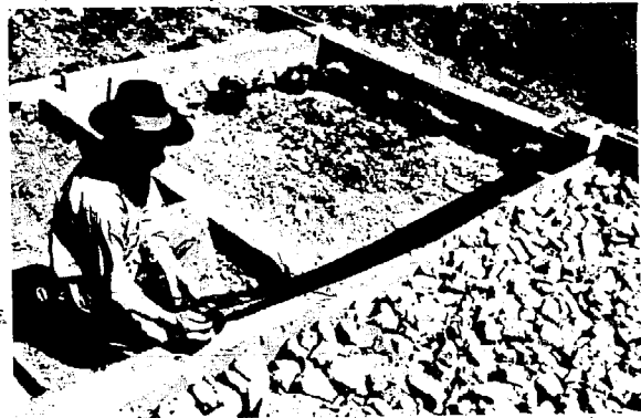
Fig. 55 Damp course of bituminous felt.
