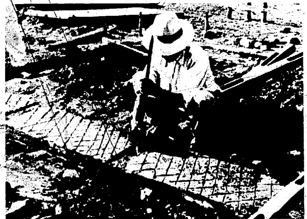
Fig. 53 Upper foundation of rammed soil-cement.
