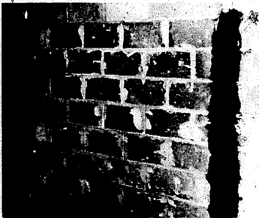
Fig. 90 Point of reference and "guide strip" for plastering a wall.
