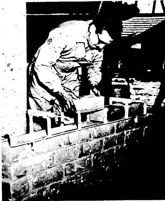
Fig. 58 Laying soil-cement blocks with a "block fitter".
