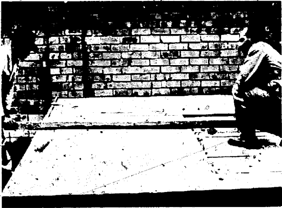
Fig. 79 Compacting the layer of soil-cement.
