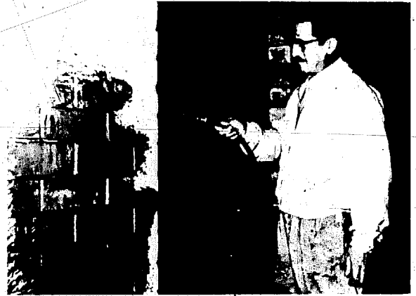
Fig. 88 Spraying a wall with water before painting.
