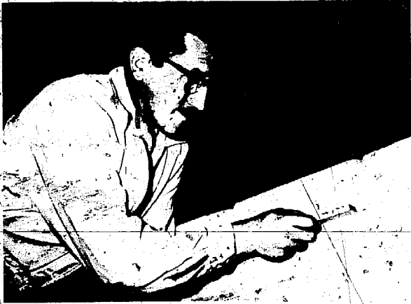
Fig. 62 Finishing an outer wall surface and trimming the seams.
