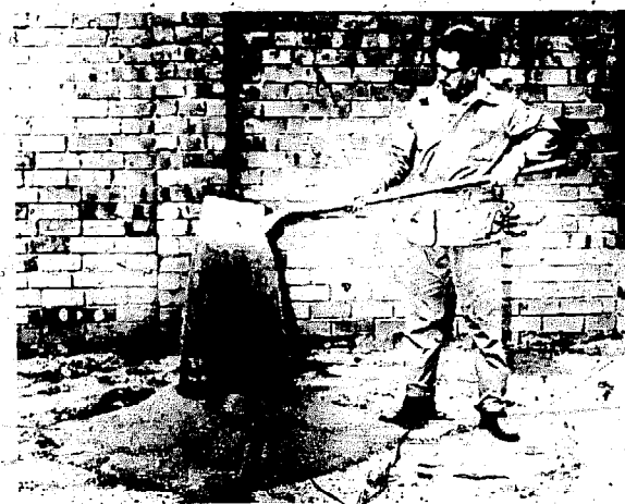
Fig. 26 Adding cement to the soil.
