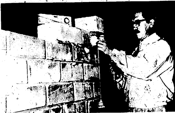
Fig. 56 Building a wall of soil-cement blocks.
