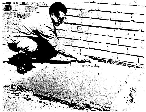
Fig. 84 (a) Smoothing the surface of a soil-cement floor with a trowel.
