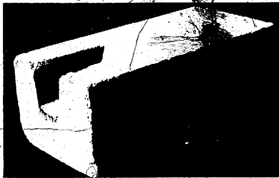
Fig. 77 Cavity block to house a dowel.
