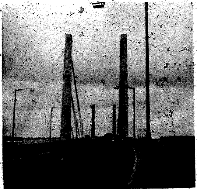
Fig 1.27 Stayed girder or cable cantilever bridge spanning the River Usk at Newport, Monmouthshire
