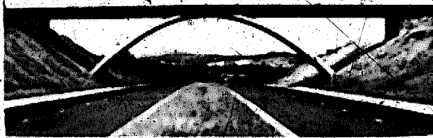
Fig 1.17 Beaconhill bridge on Ross Street Motorway
