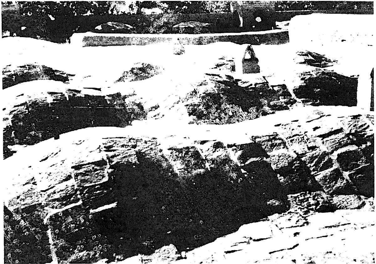
FIG. 5.25. Doubly curved mud-vault roof, Iran.
