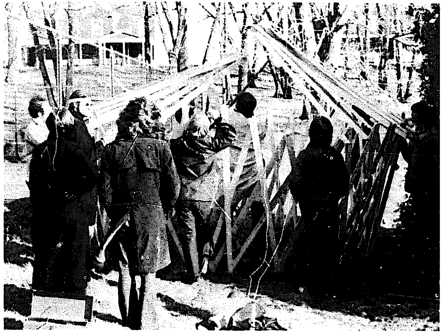
Pole method of supporting roof pieces.
