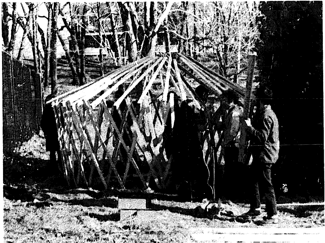
Roof assembly in progress.
